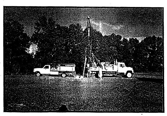
Installing groundwater monitoring wells at New River MCAS Site 48
