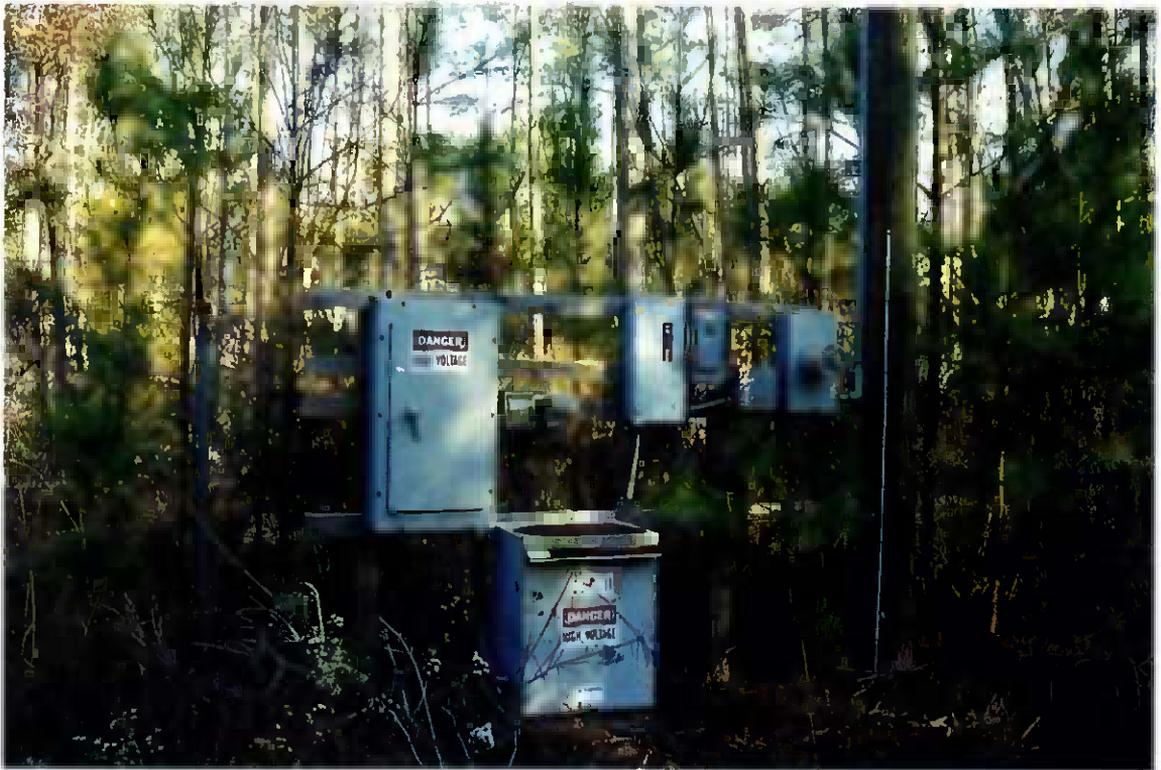
**1998. Site 69** Power cables that ran to the treatment system are still connected to the power panel outside the fence at Site 69.
