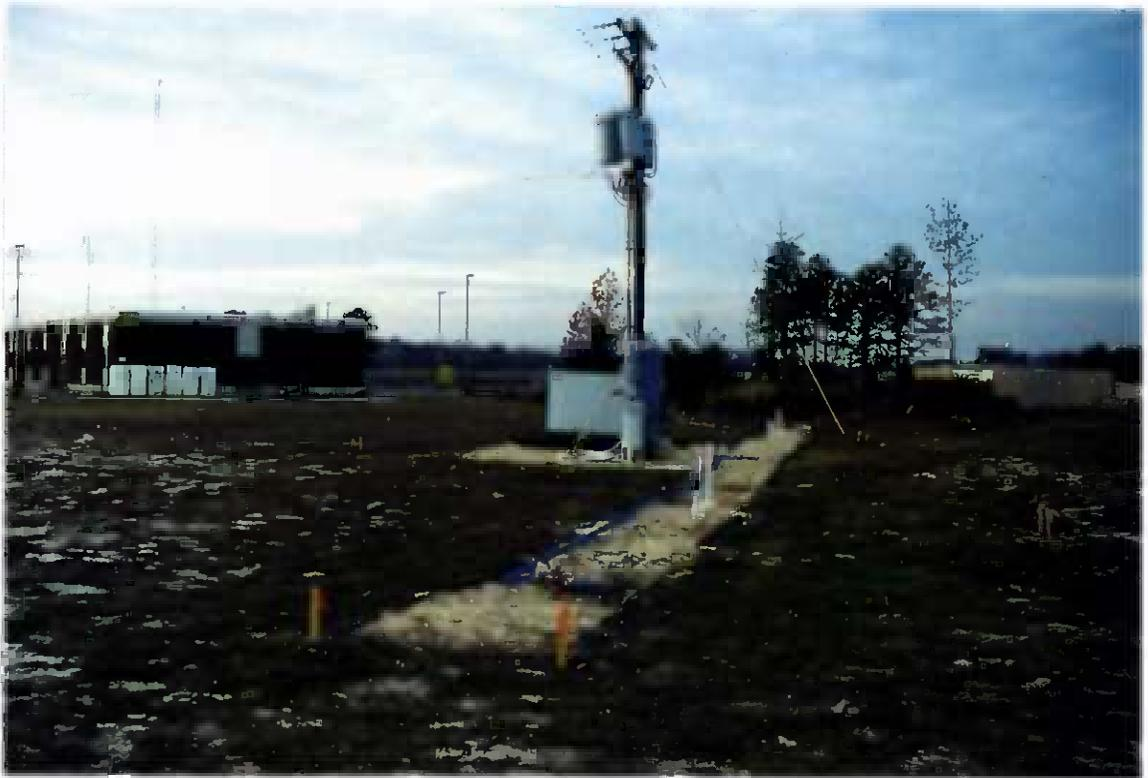
**1998. Site 35** Air sparging is currently taking place at Site 35. The air sparging trench, pictured here, will remain operational after the U.S. Highway 17 bypass is complete.
