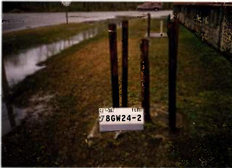
**Figure 4-3** Intermediate monitoring well 78-GW24-2 was constructed during the 1986 Confirmation Study without a locking cap.
