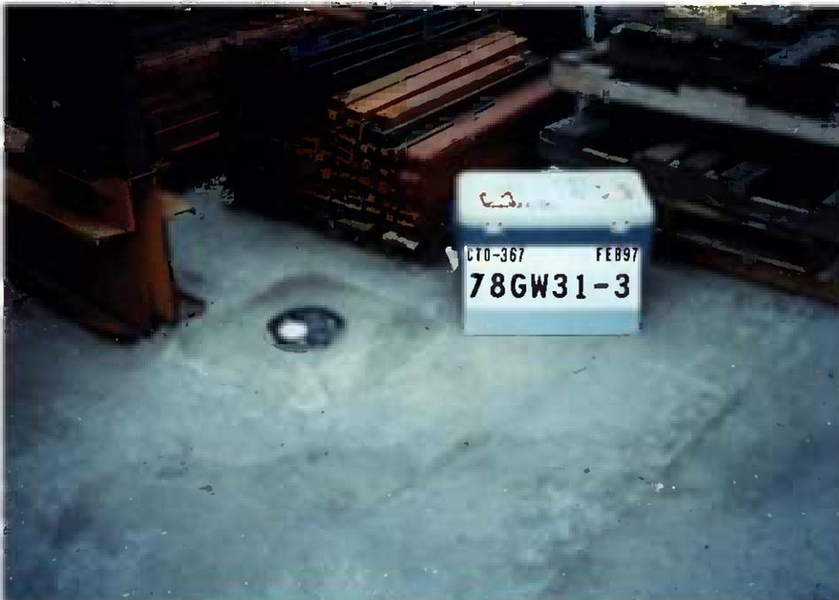
**Figure 4-6** A new protective cover and concrete pad were installed at deep well 78-GW31-3. The new concrete pad was constructed with a slightly higher elevation so that runoff would be less likely to enter the well.
