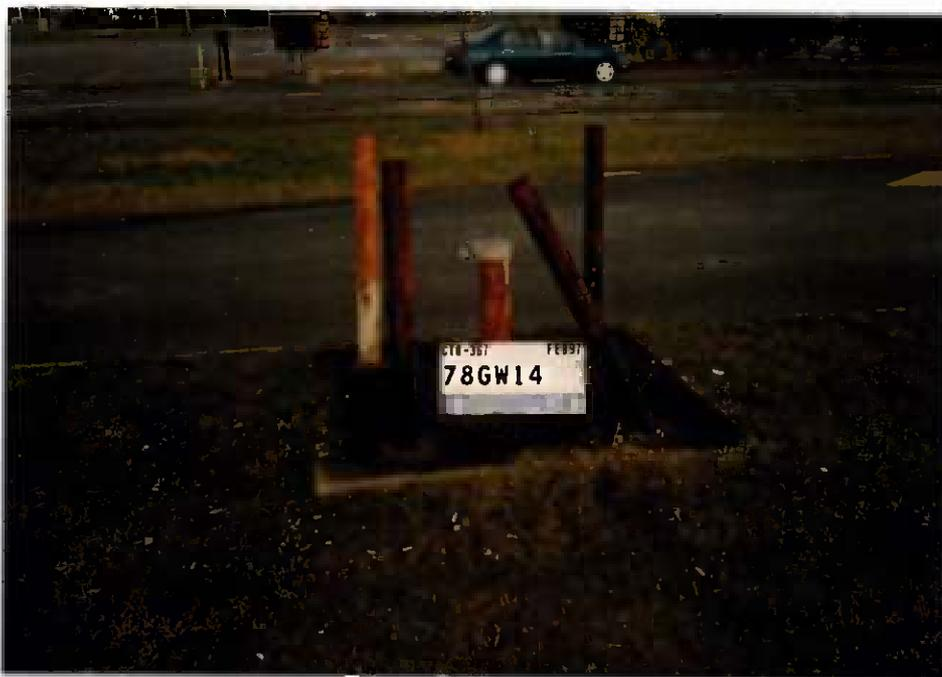
**Figure 4-9** Shallow monitoring well 78-GW14 is located in a high-traffic area. One of the four protective bollards had been recently struck by a vehicle and bent.
