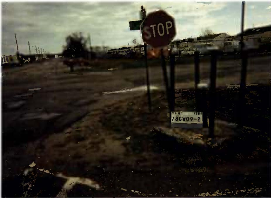
**Figure 4-7** Soil from beneath the pad of intermediate monitoring well 78-GW09-2 had begun to erode and the well had become unsightly.
