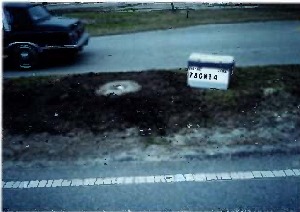
**Figure 4-10** Monitoring well 78-GW14 was converted from a stick-up to a flush mount to reduce the possibility of damage from further collisions. Top soil and grass seed were used to restore the site.
