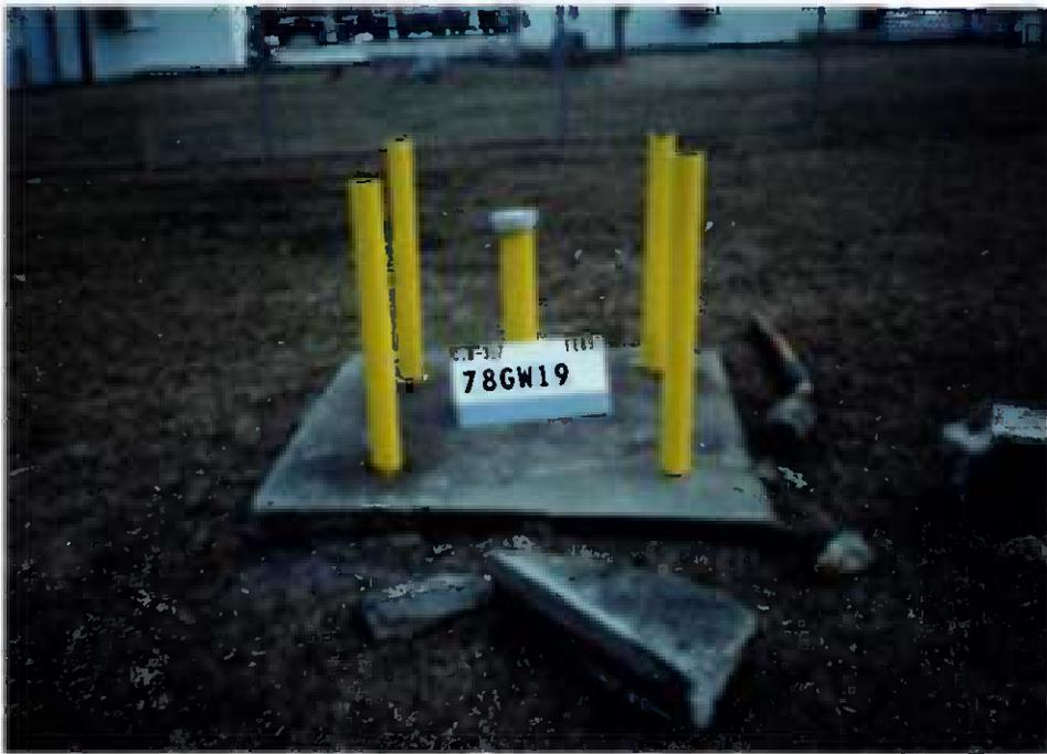
**Figure 4-12** The damaged bollard was replaced and the concrete pad of well 78-GW19 was repaired. The excess concrete and bollard, pictured here, were removed after all well maintenance activities had been completed.
