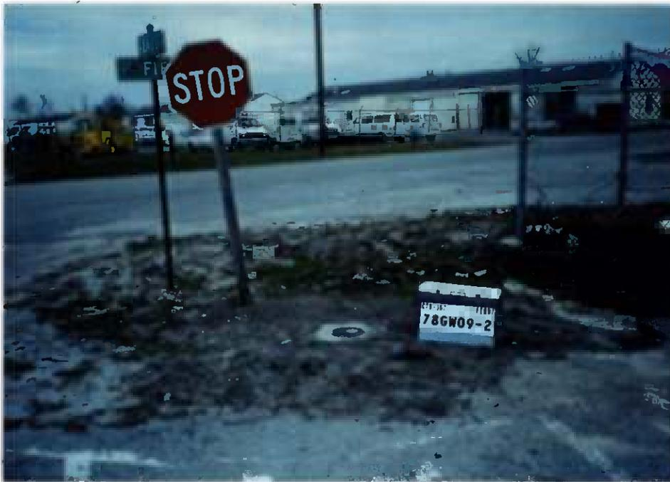
**Figure 4-8** Monitoring well 78-GW09-2 was converted from a stick-up to a flush mount. Topsoil and grass seed were used to restore the site.
