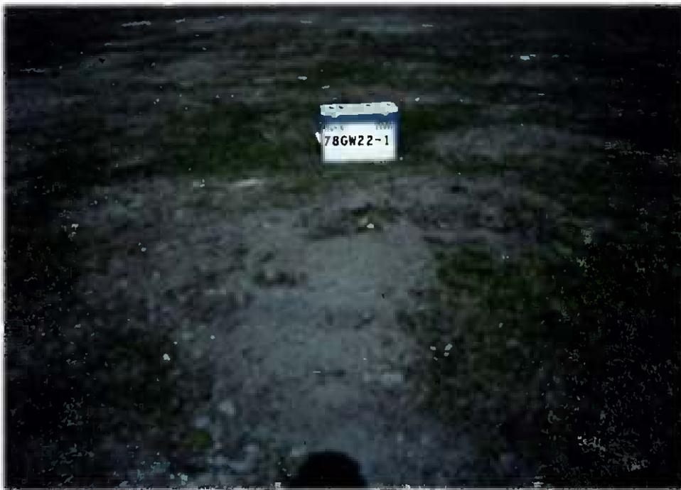
**Figure 4-2** The pad, bollards, and protective casing of monitoring well 78-GW22-1 were also removed. Topsoil and grass seed were used to restore the site.
