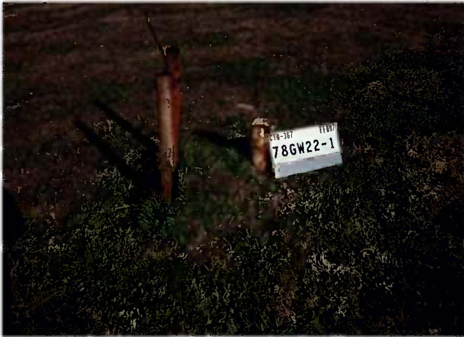
**Figure 4-1** Shallow monitoring well 78-GW22-1 was abandoned according to procedures stipulated by North Carolina. The well had begun to exhibit signs of subsurface deterioration.
