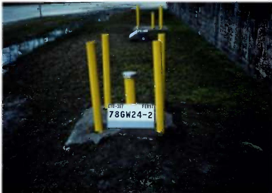
**Figure 4-4** A locking cap and lock were installed on monitoring well 78-GW24-2. In addition, peeling paint and rust were removed and two coats of paint were then applied.
