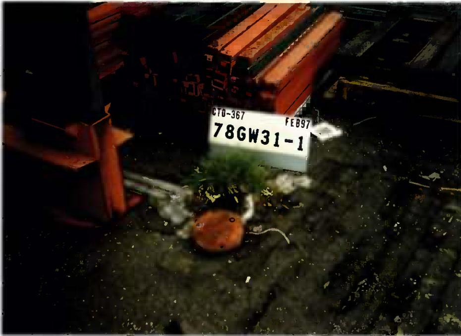
**Figure 4-5** The protective lid of deep monitoring well 78-GW31-3 was damaged. Without a proper seal runoff from the surrounding parking area may have entered the well.
