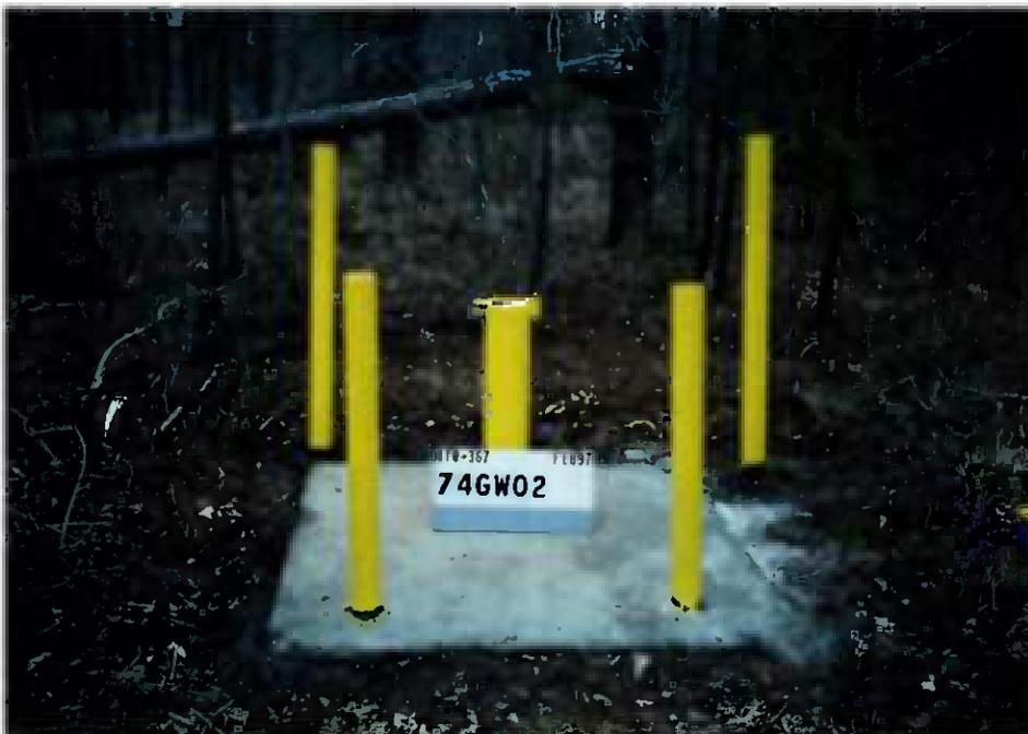
**Figure 3-4** The bollards and protective casing of monitoring well 74-GW02 were first scraped to remove peeling paint and rust, and then weather resistant paint was applied. New padlocks were also installed on each of the Site 74 monitoring wells.
