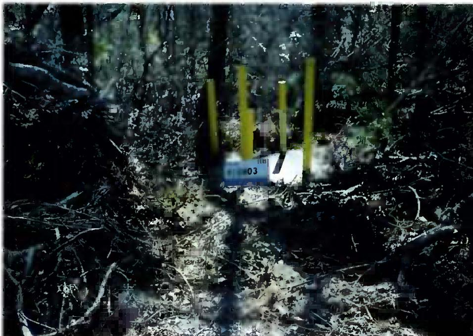
**Figure 3-2** The downed trees were removed from atop the well and an access path was cleared. Weather resistant paint was then applied to the bollards and protective casing of well 41-GW03.
