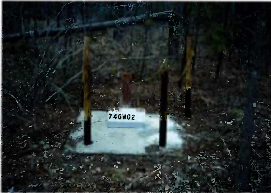
**Figure 3-3** Shallow monitoring well 74-GW02 was constructed during the 1984 Confirmation Study. The well had begun to exhibit signs of deterioration.
