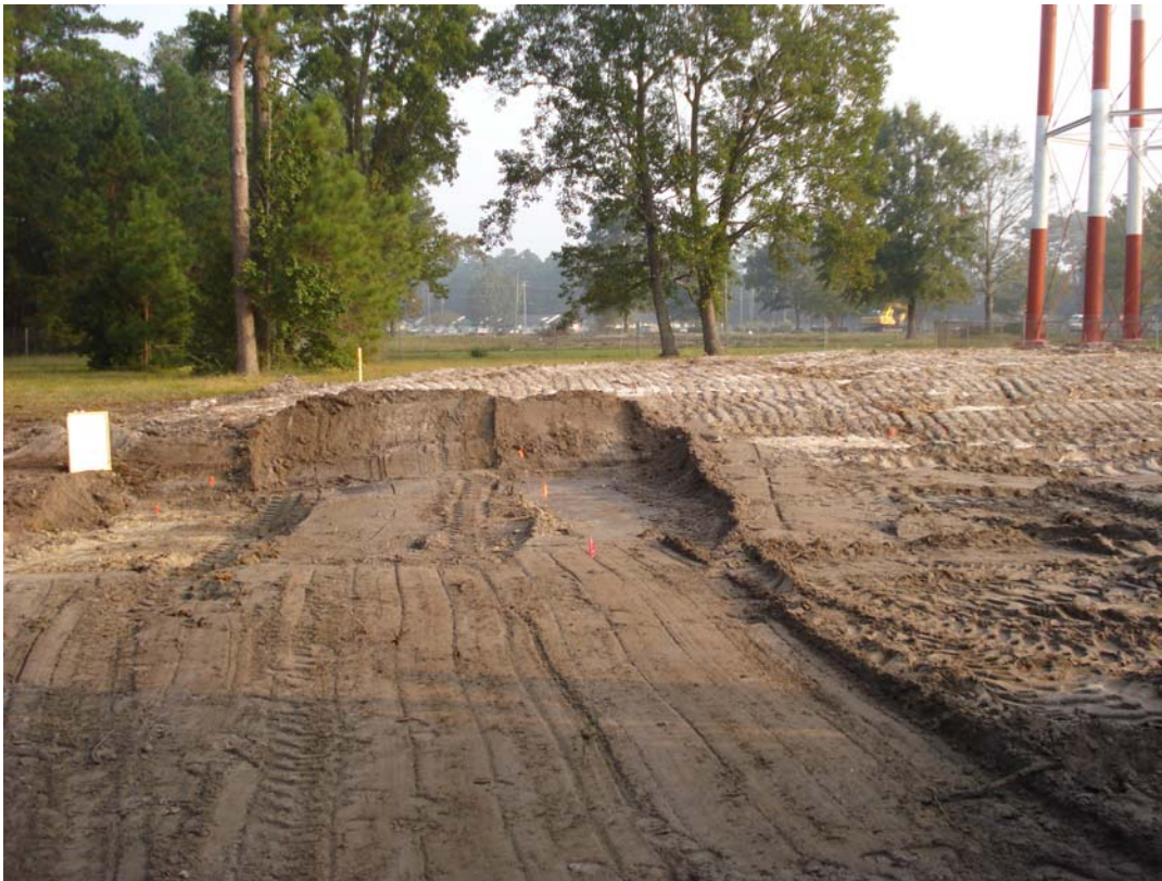
Surface Release area excavation with sample flags
