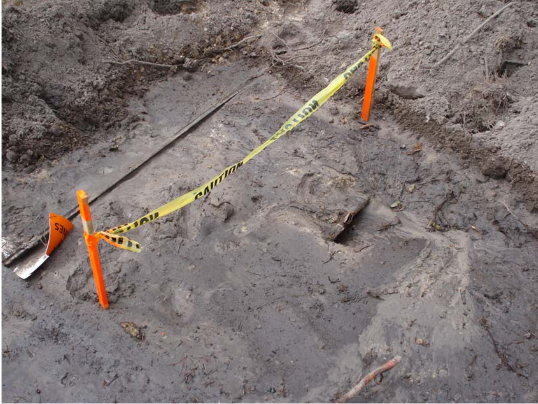
Tank TT-2778 prior to removal
