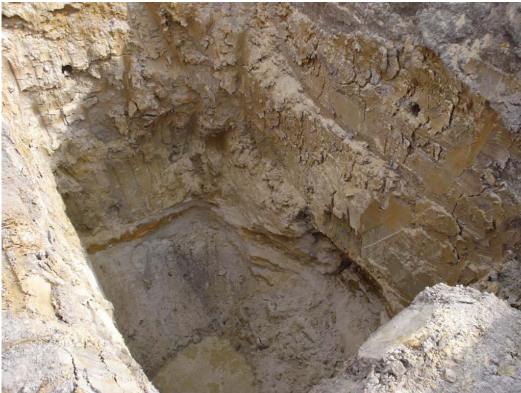
Final excavation of TT-2778 tank basin
