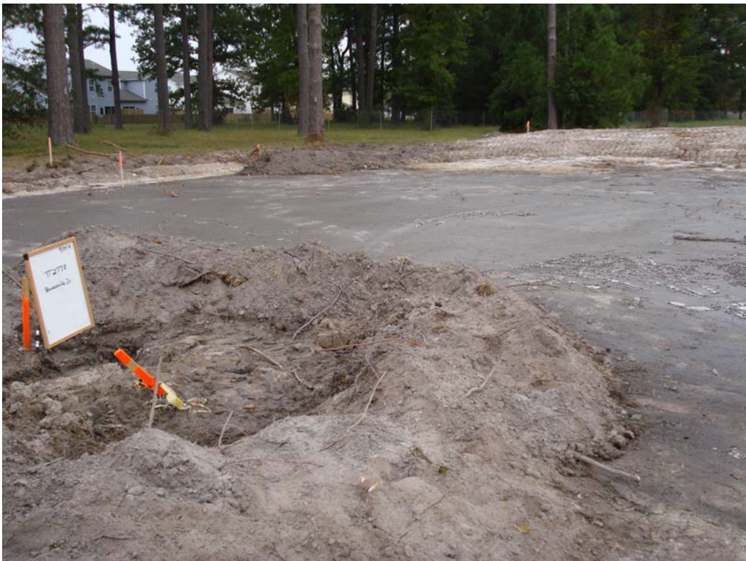
TT-2778 prior to removal
