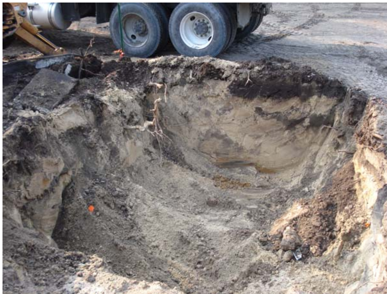
Excavation activities – Looking south
