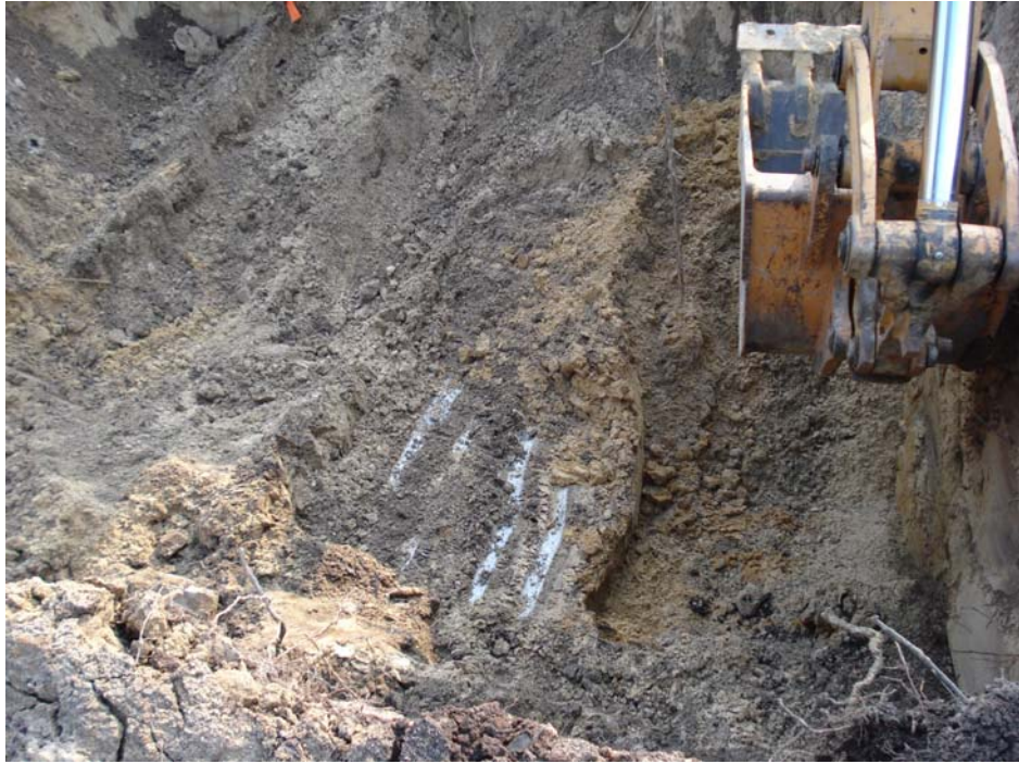
Bottom of excavation – concrete pad
