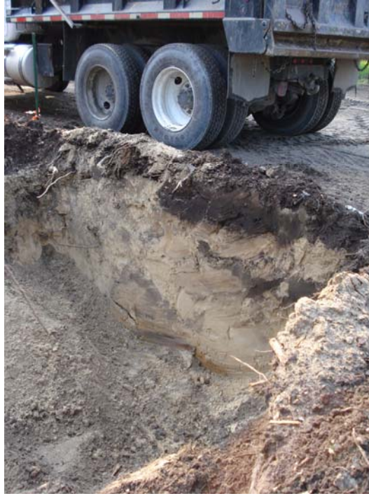
Excavation activities – south wall
