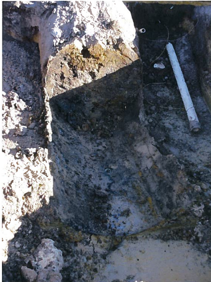
TT-3127 tank basin immediately after removal of UST
