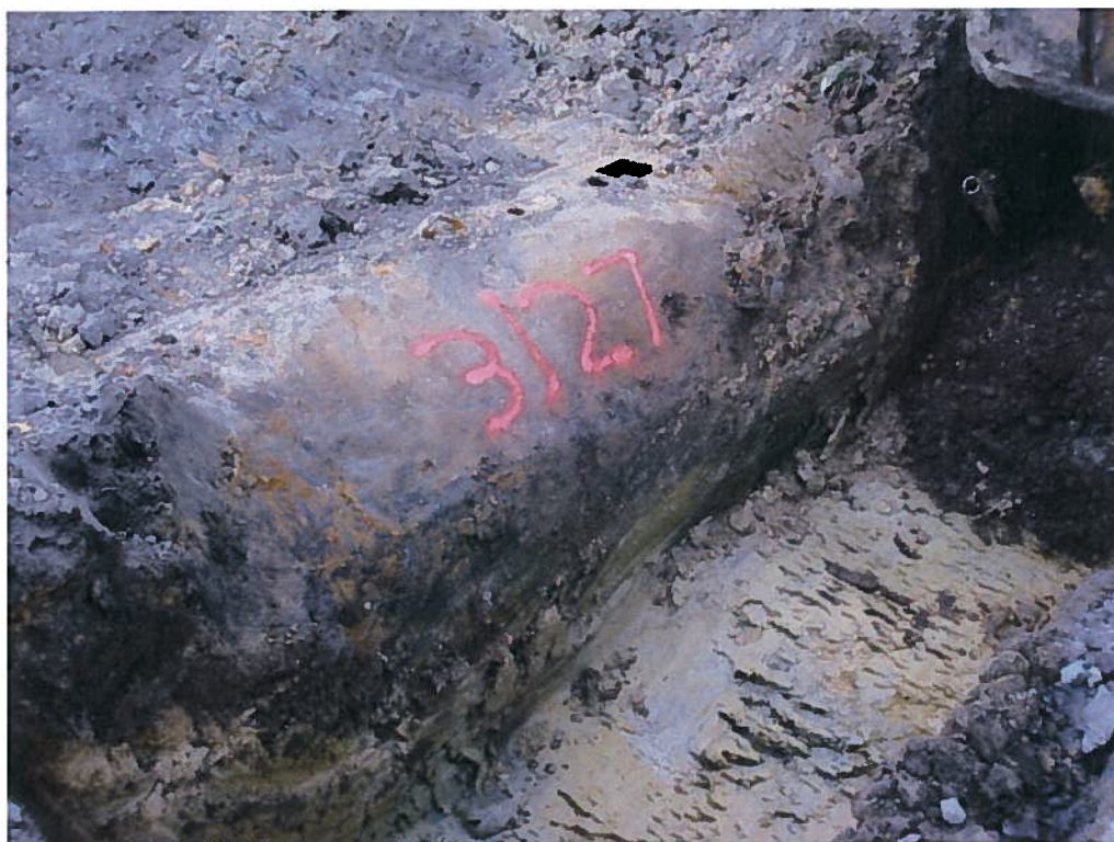
UST TT-3127 prior to removal with access hole
