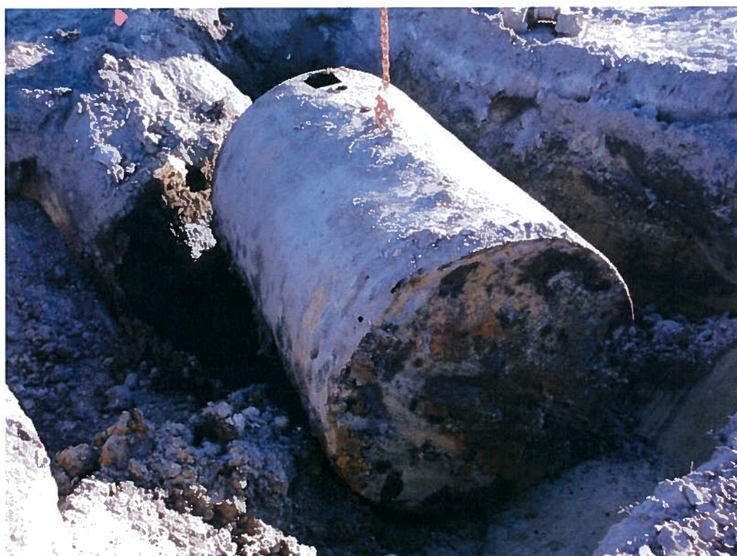
UST TT-3127 during removal activities
