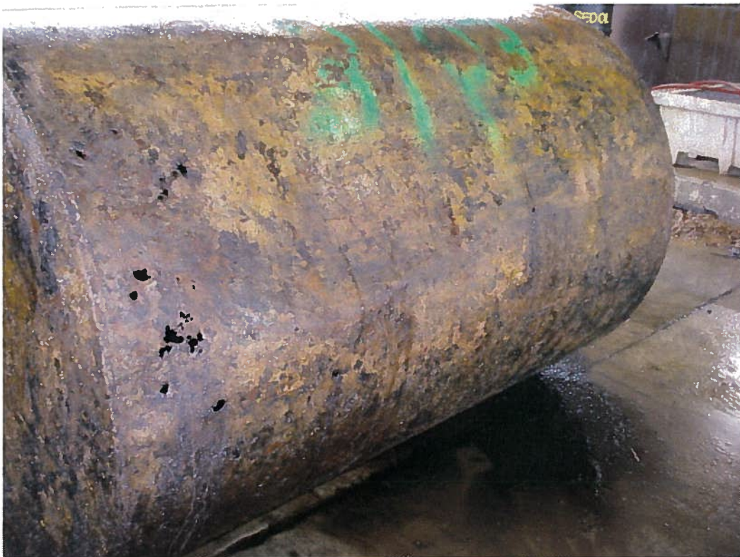
UST TT-3103 after cleaning at RCRS, Building 977
