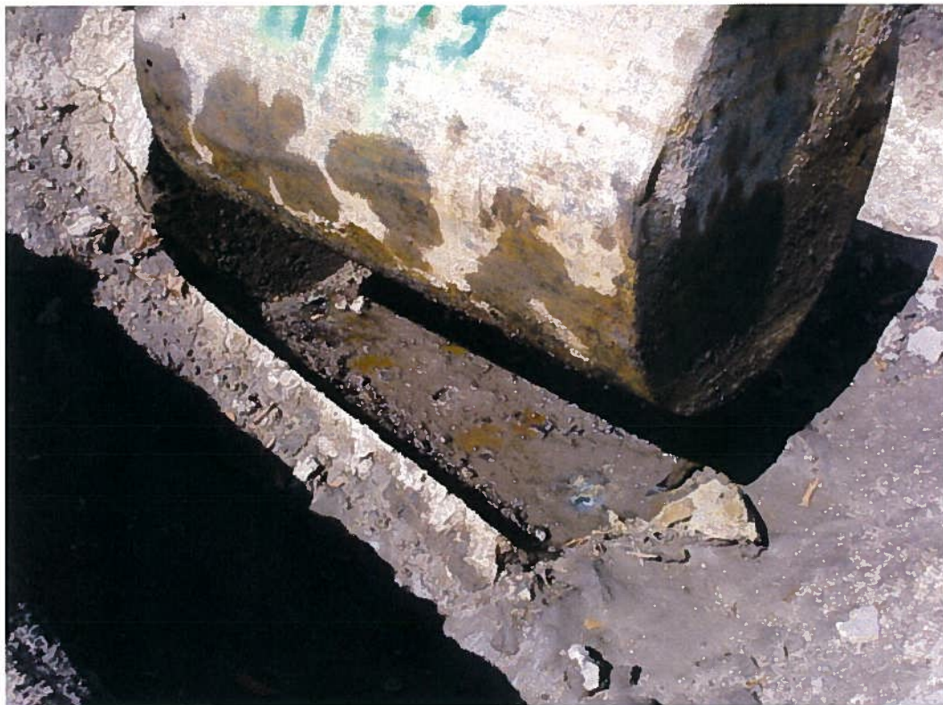
UST TT-3103 during removal activities
