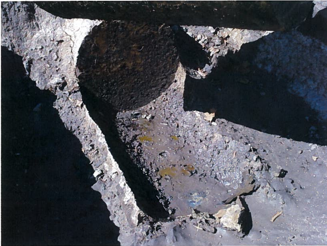
TT-3103 tank basin immediately after removal of UST
