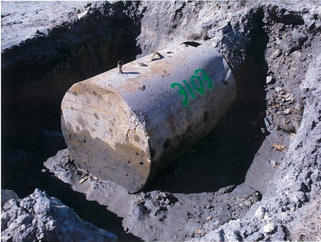
UST TT-3103 prior to removal with access hole
