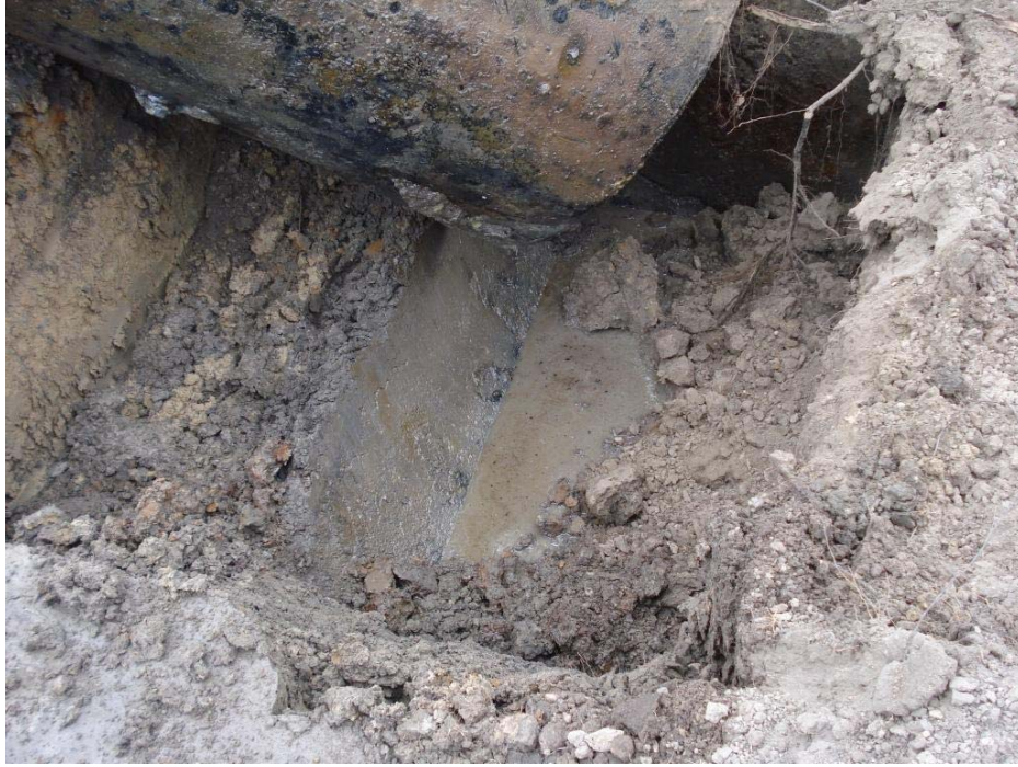
TT-2361 tank removal
