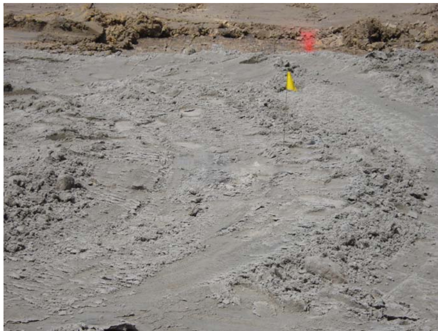
TT2223 Backfilled Excavation with Temporary Monitoring Well Location.
