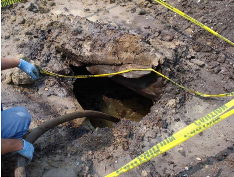
TT2223 Residual Pumping prior to Excavation.
