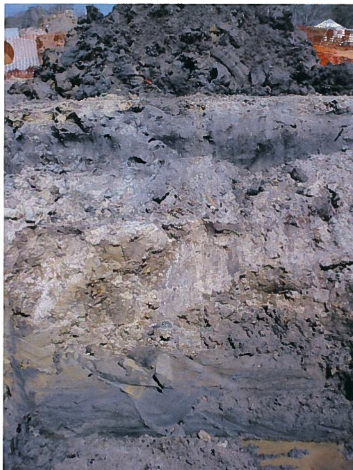
Final depth of excavation at UST TT-2084
