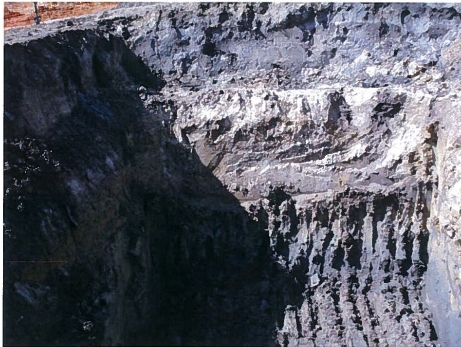
Excavation after removal of UST TT-2084
