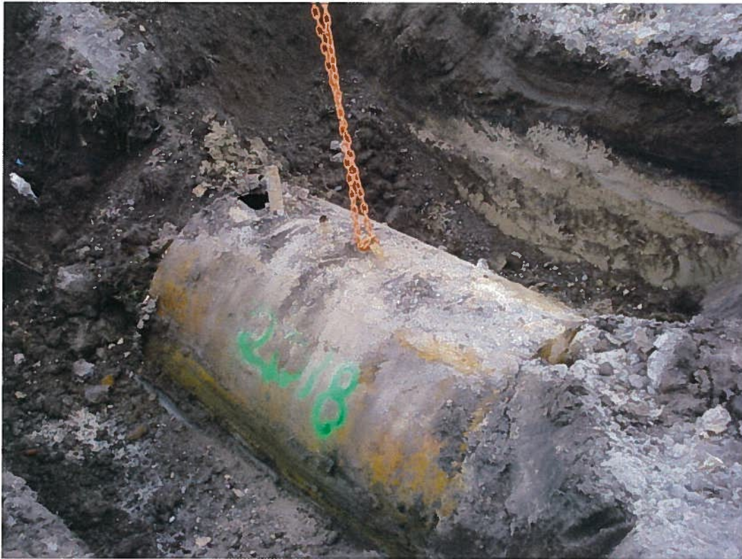
UST TT-2018 prior to removal with access hole
