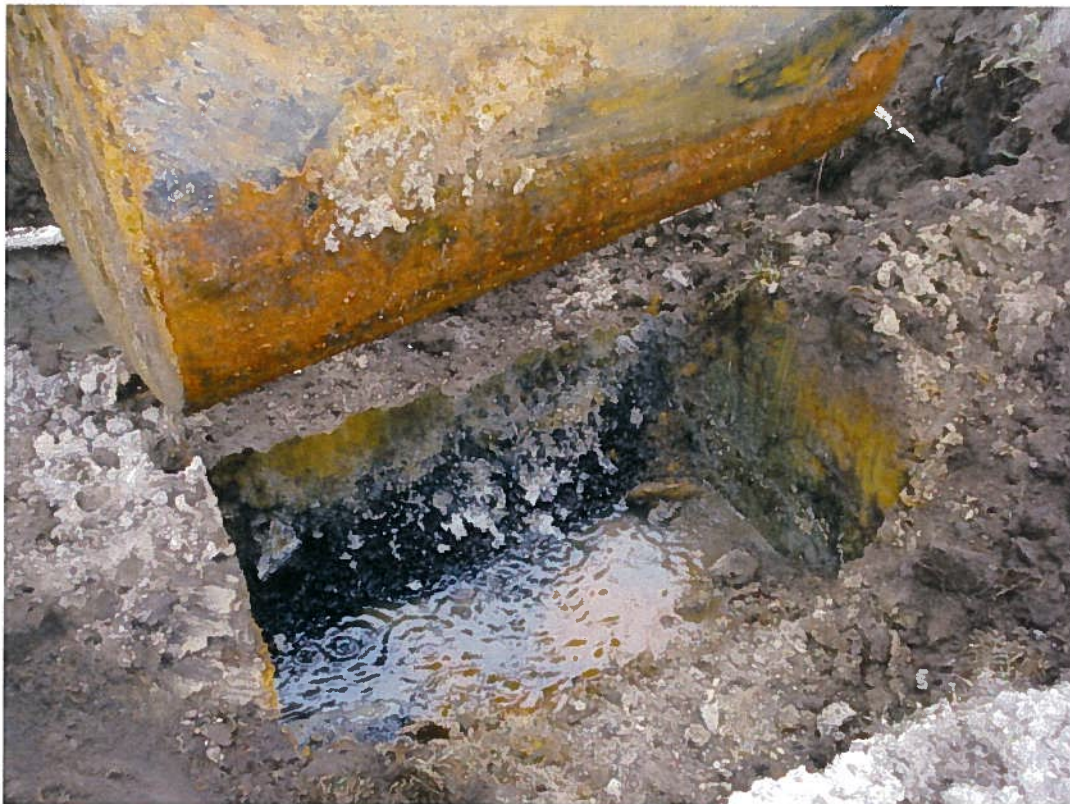
UST TT-2018 during removal activities
