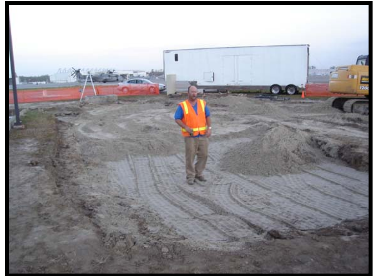
Backfill at tracer probes 196, 200 & 201
