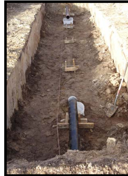
Removed leaking pipe sections at tracer probe 184 & 185
