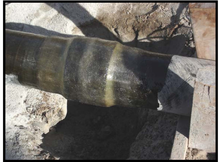
Coupling between existing and new pipe sections
