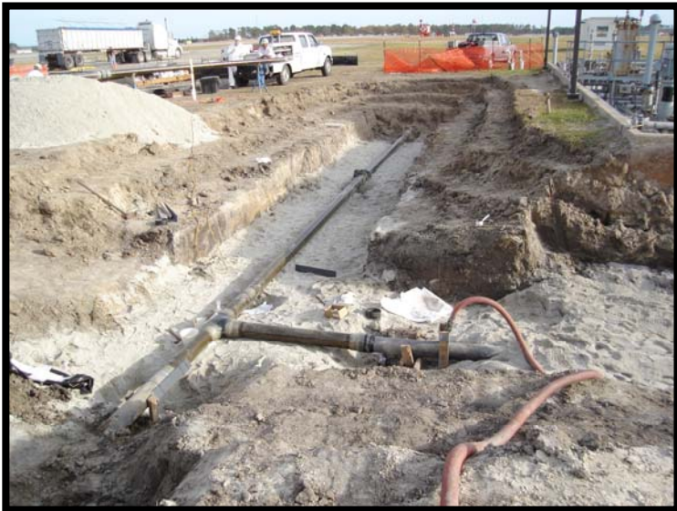
New pipe section at tracer probes 196, 200 & 201
