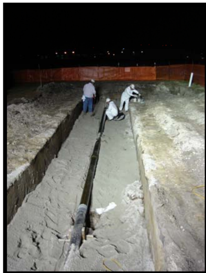
New pipe sections at tracer probes 184 & 185
