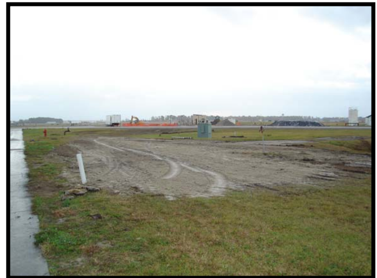
Backfilled pipe at tracer location 184 & 185
