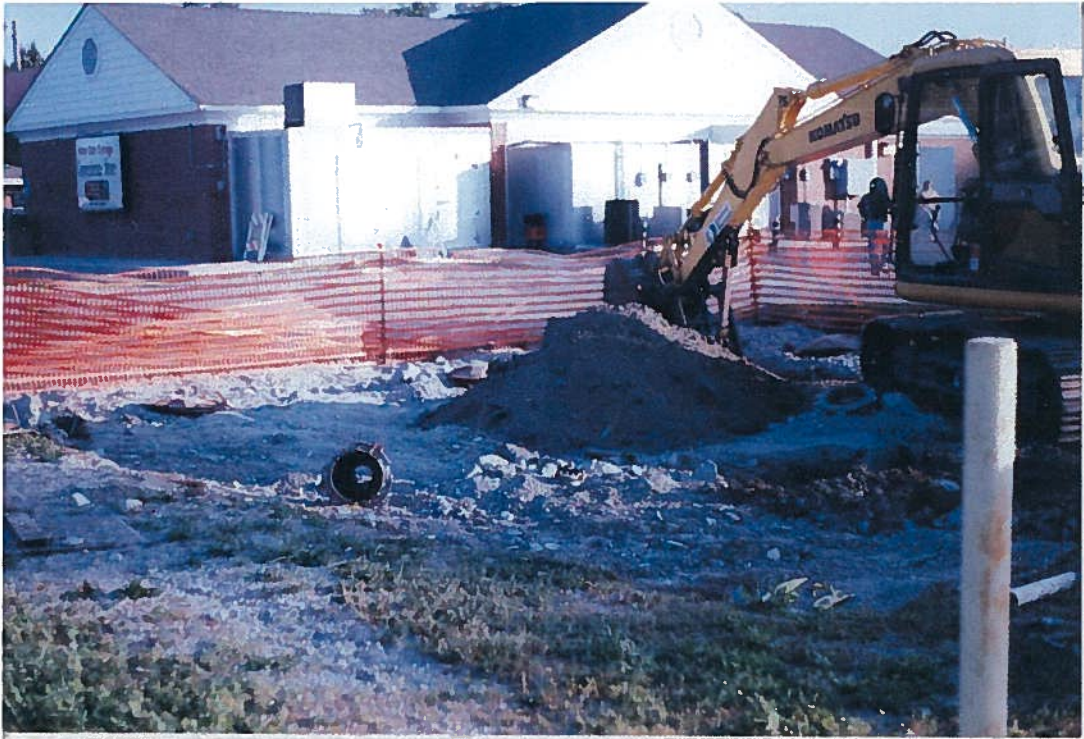
Photo #1 Excavating to Expose tanks.
