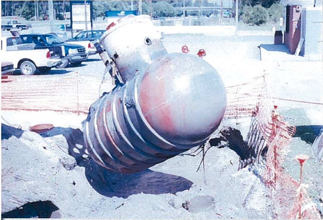
Photo #3 UST LCH 4034-3 (2,500-gallon) removed out of ground.
