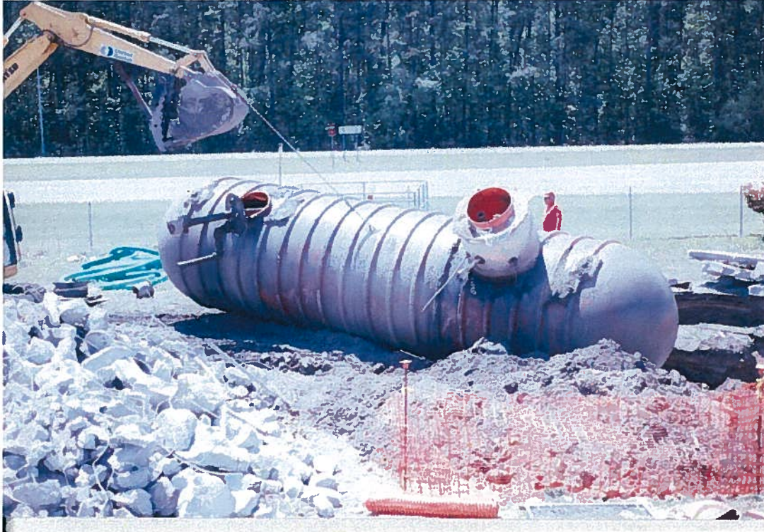
Photo #5 UST LCH 4034-1 (10,000-gallon) removed out of ground.
