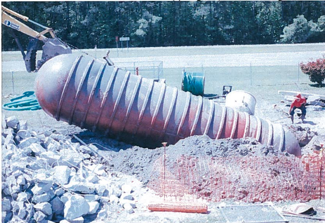
Photo #4 UST LCH 4034-2 (10,000-gallon) removed out of ground.
