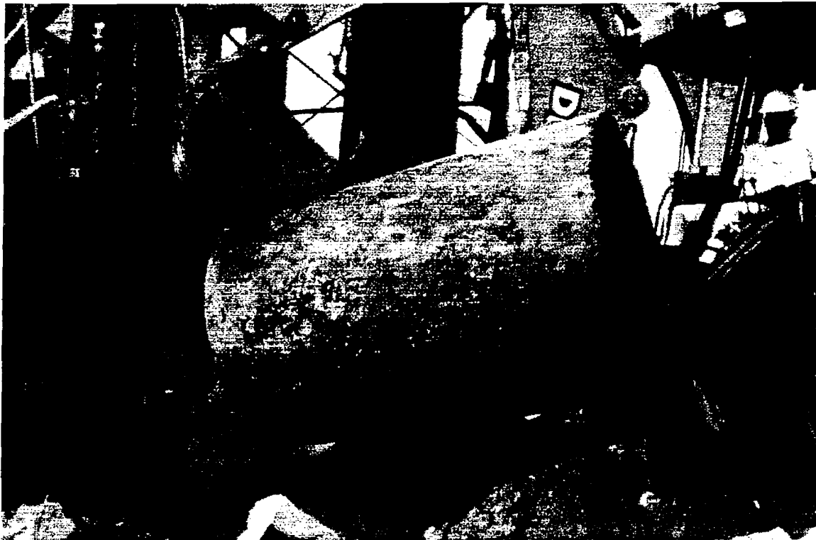
Photo 5 UST Removal Activities There are not any rust holes or oily appearances on the tank.
