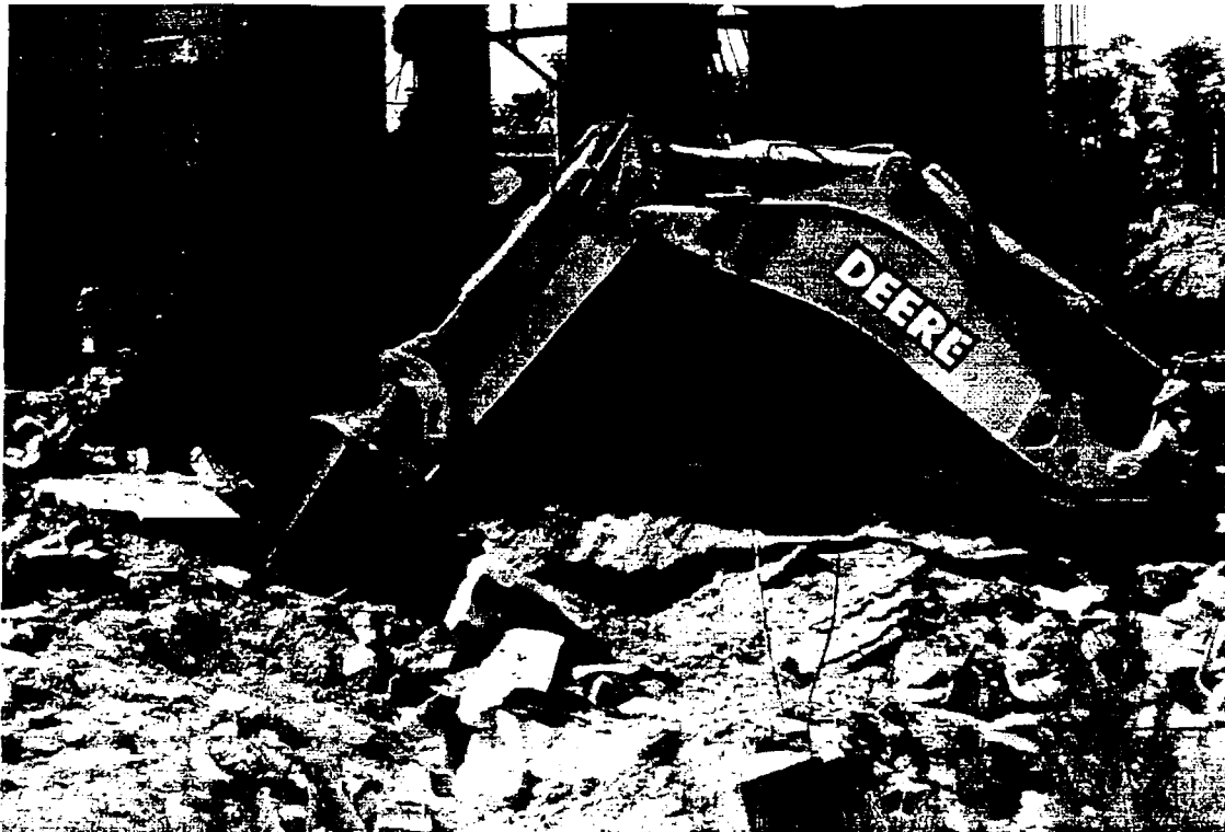
Photo 9 8/5/99 Site Undergoing Over-Excavation Debris and rubble over excavation placed by others.
