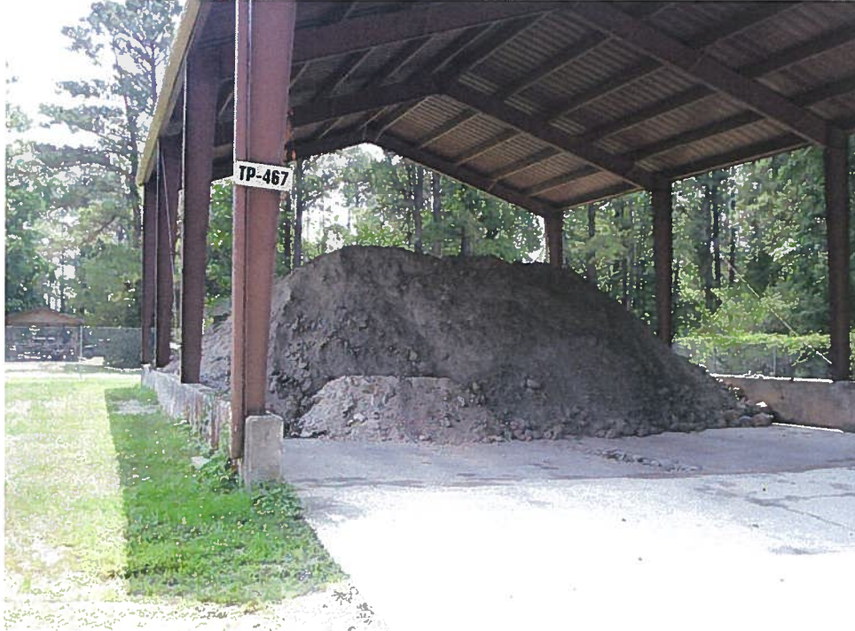
Photo 5; TP-467 Soil stockpile drying pad (front view).
