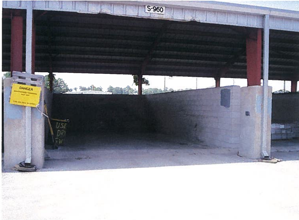
Photo 3; S-960 Soil stockpile drying pad after 52.52 Tons soil removed.
