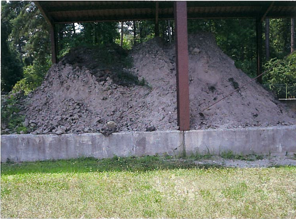
Photo 6; TP-467 Soil stockpile drying pad (side view).
