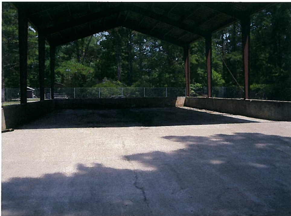
Photo 8; TP-467 Project conclusion. Soil stockpile drying pad left "broom clean".
