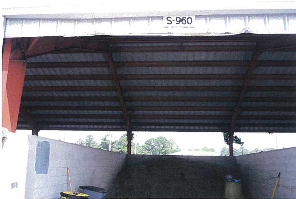
Photo 1; S-960 Soil stockpile drying pad
