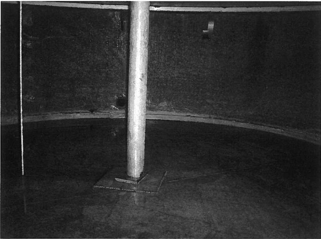
Photo 14: Lower portion of AST after cleaning completed.
