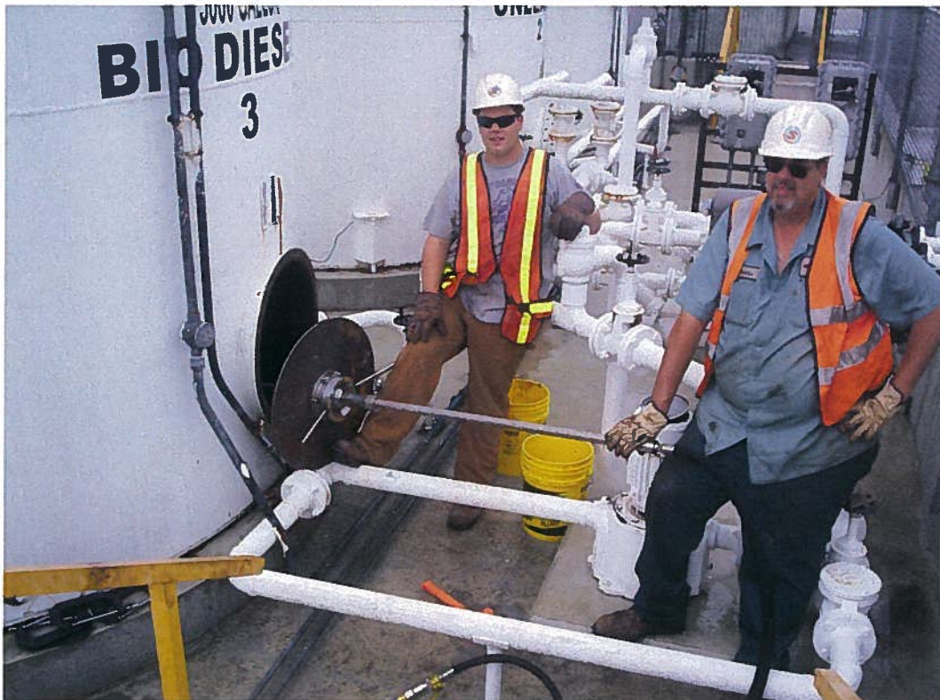
Photo 9; Final preparations for cleaning lower portion of AST.
