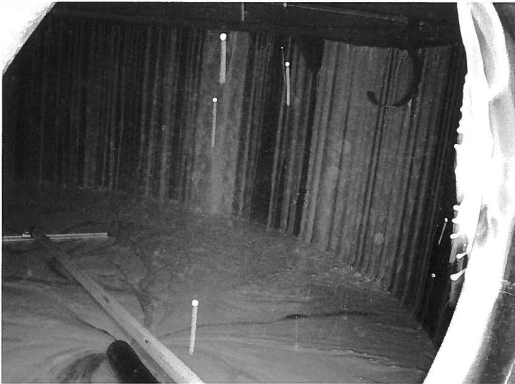
Photo 13: Triple application of cleaning solution in progress.
