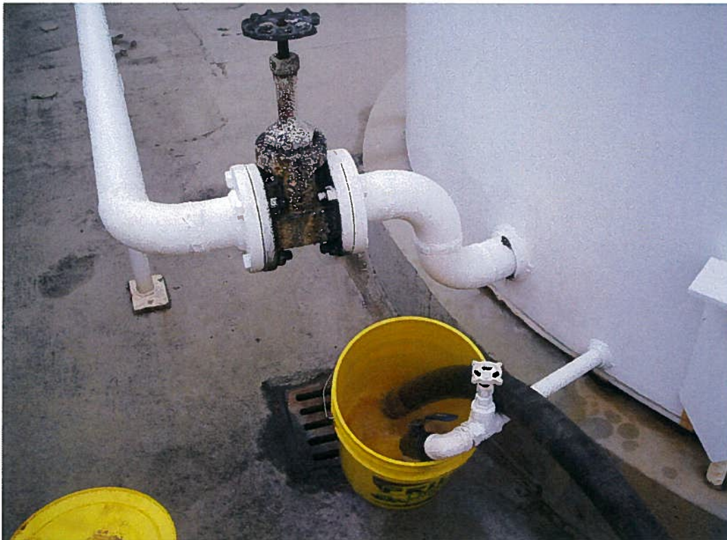
Photo 2; Decanting nuisance water from bottom of tank for disposal at EMD.
