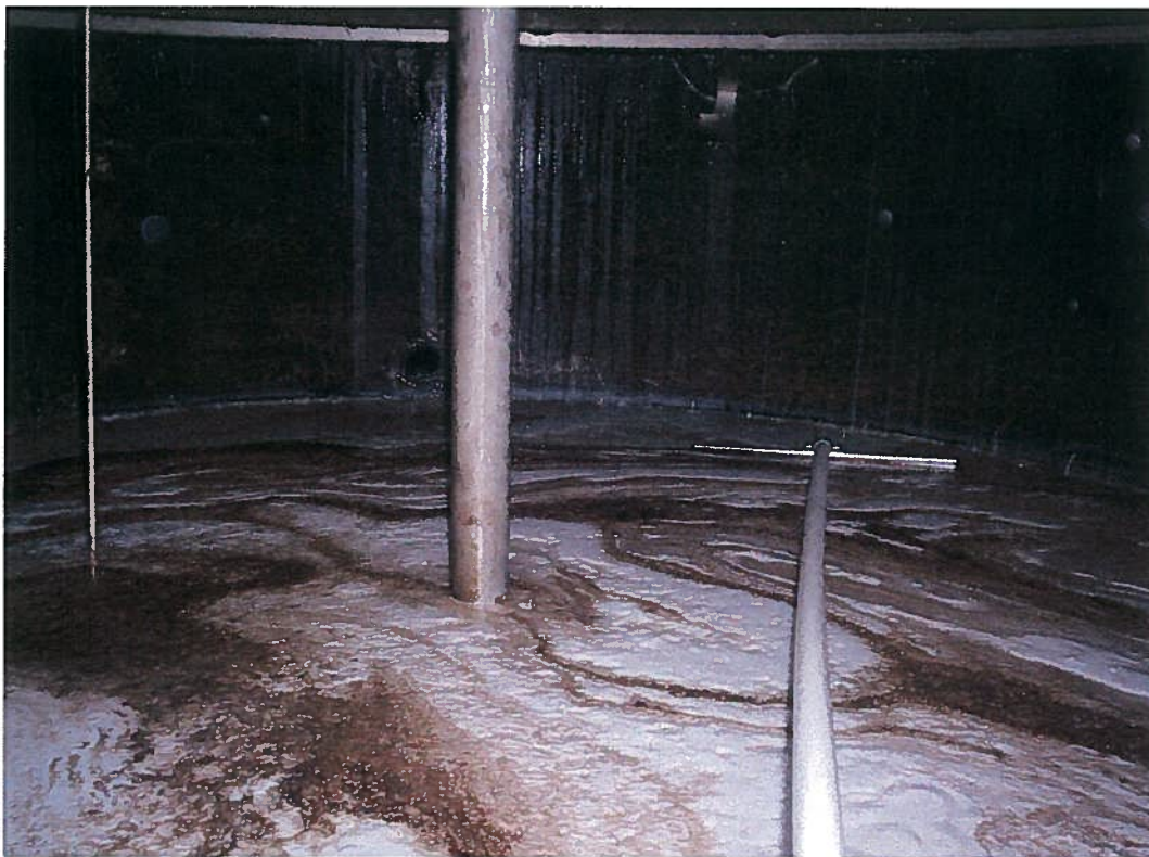
Photo 12; Emulsification of residual bio-diesel and cleaning solution.
