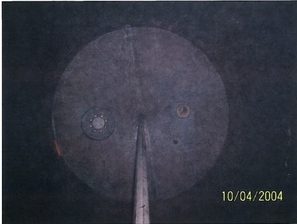
Underside of the Fixed Roof
