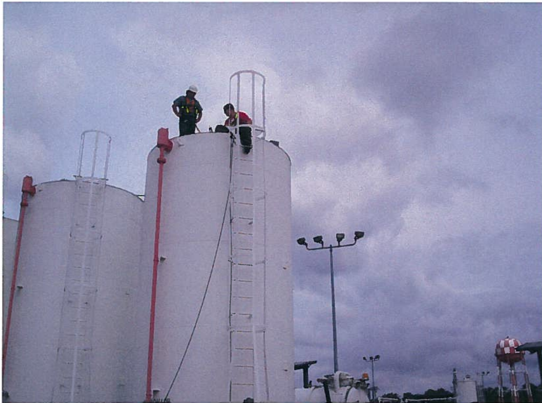
Photo 10; Gaining access to upper portion of AST for cleaning.
