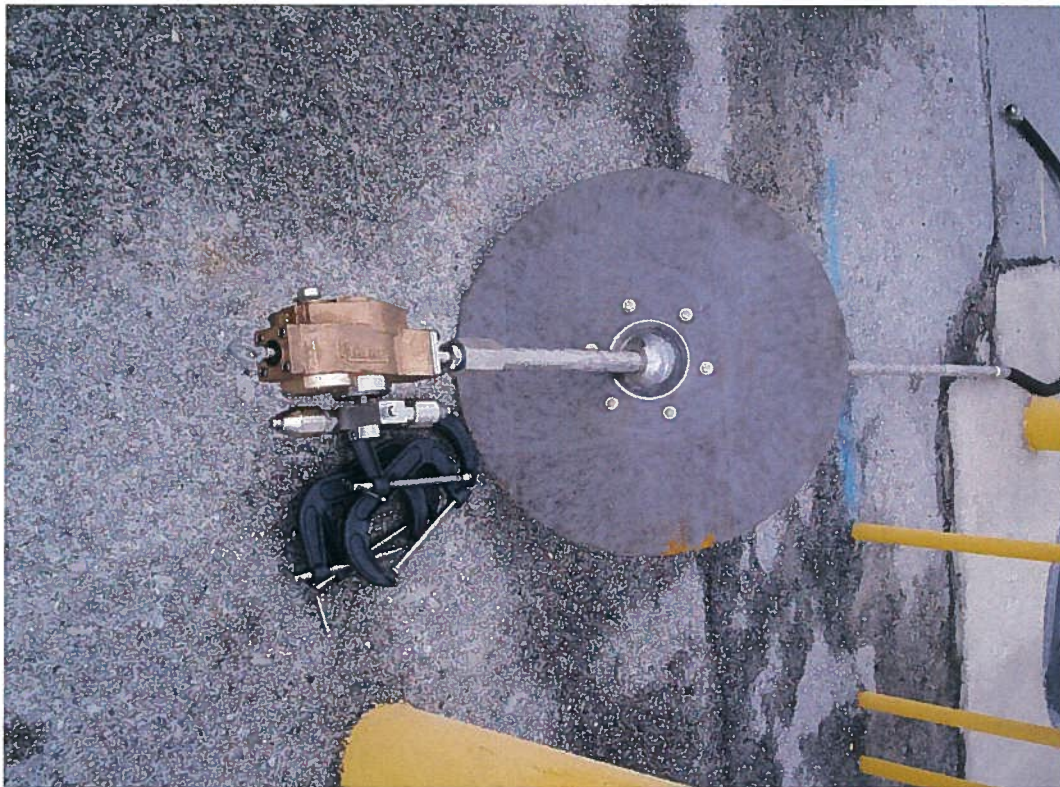
Photo 8: Man way mounting plate and spray nozzle assembly.
