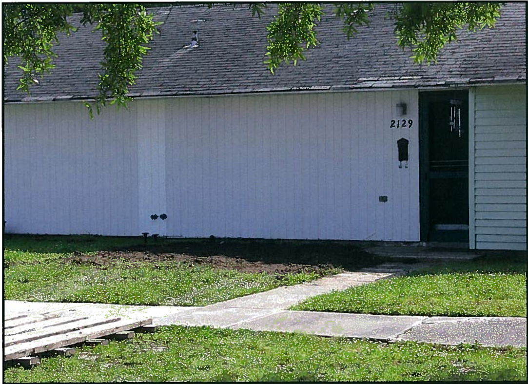
UST TT-2129 following soil removal and backfilling
