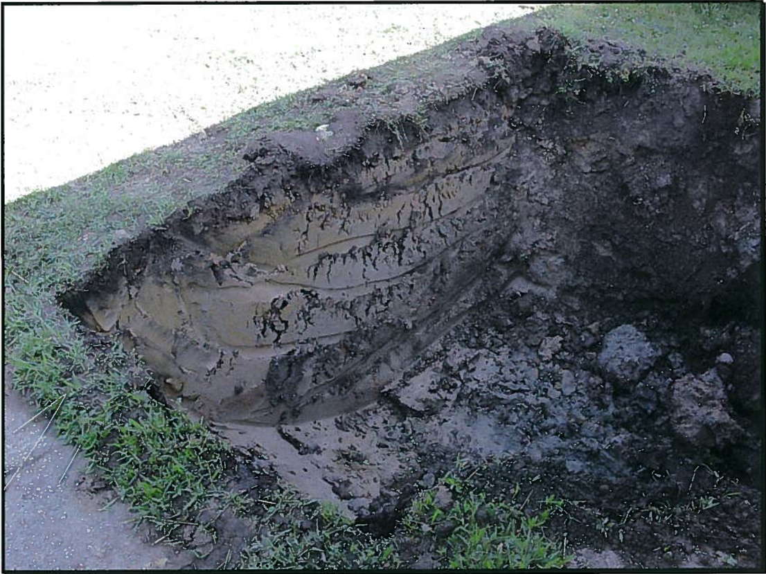
UST TT-2129 soil excavation
