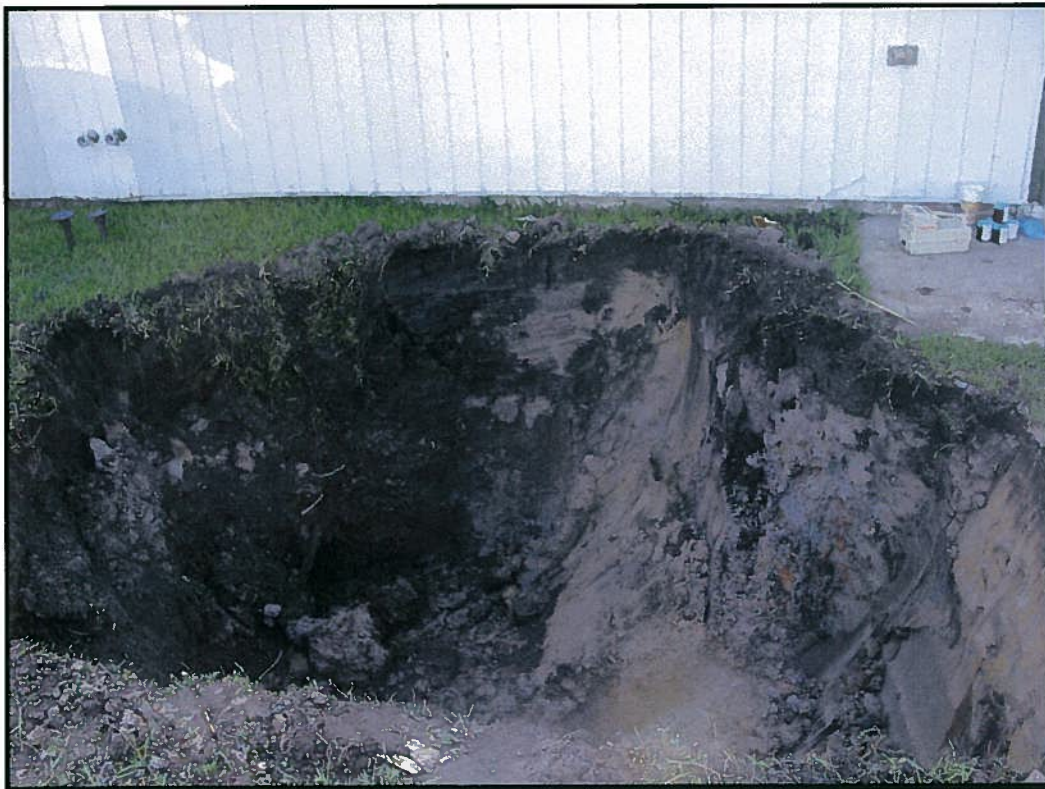
UST TT-2129 soil removal activities
