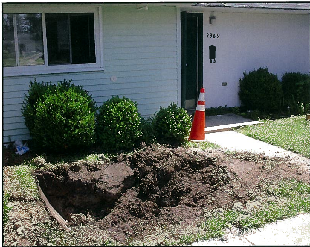
Former UST TT-2969 location
