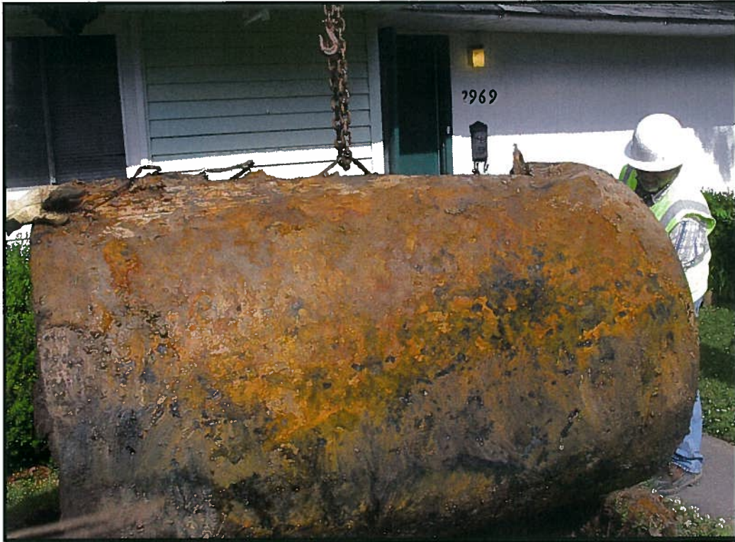
Removed UST TT-2969
