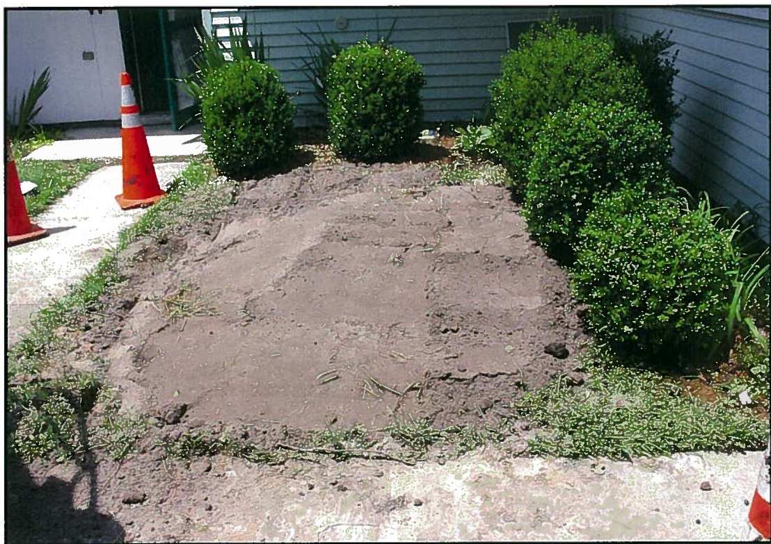
Backfilled former UST TT-2969 location
