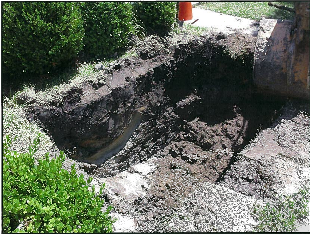
UST TT-2969 soil removal activities
