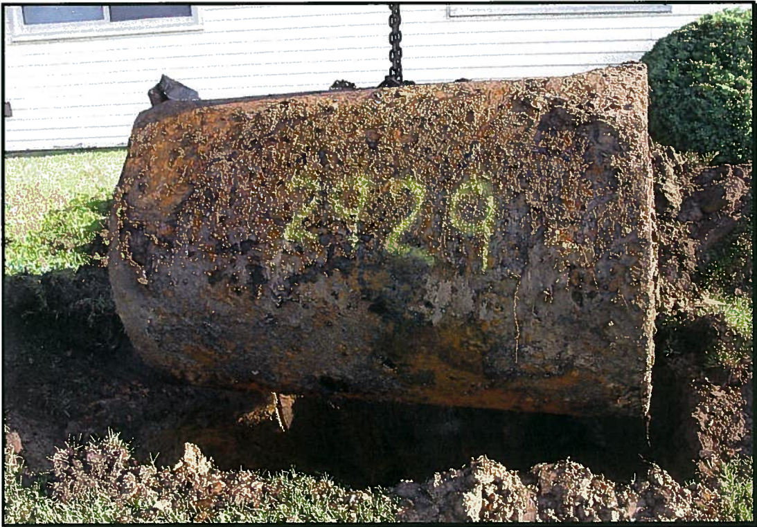
Removed UST TT-2929
