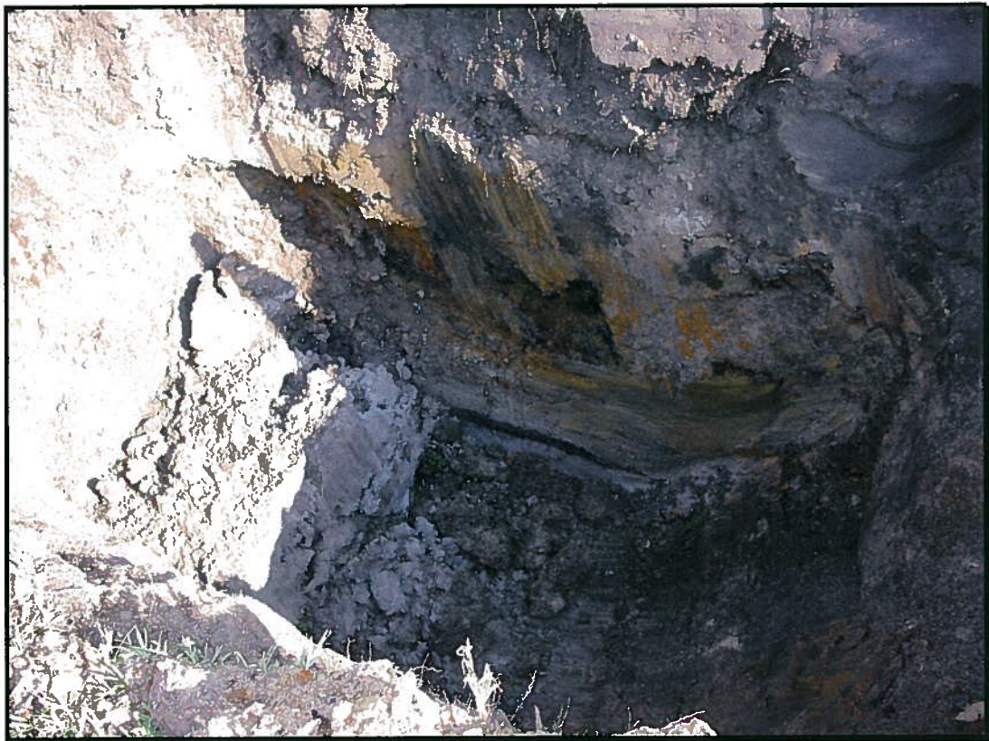
UST TT-2929 soil removal activities
