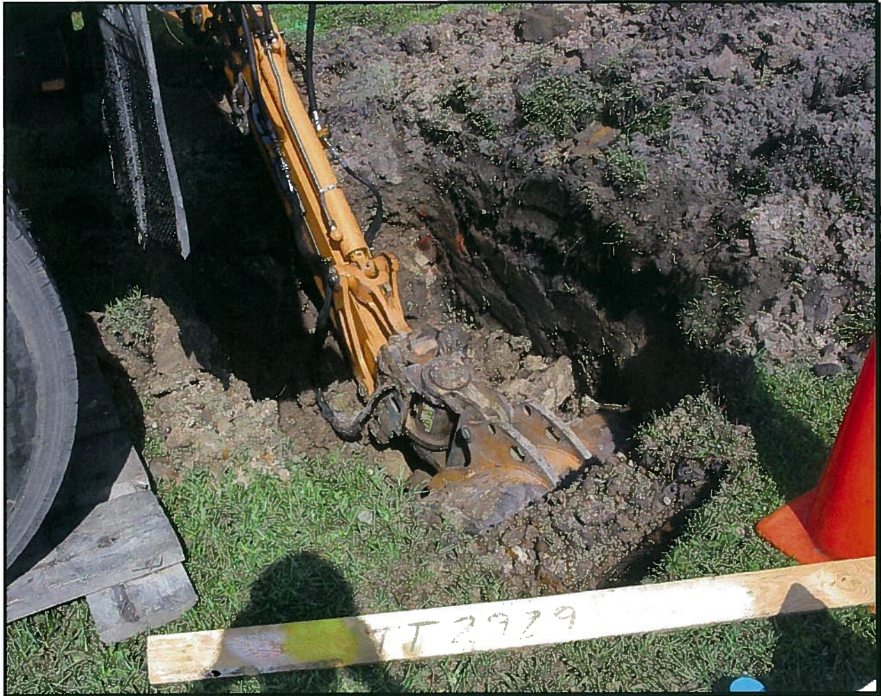
UST TT-2929 soil removal activities
