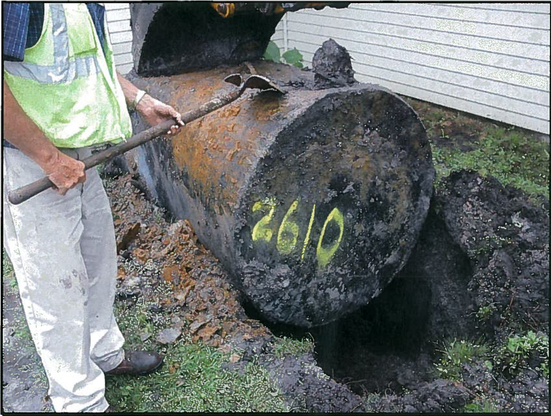
UST TT-2610 during removal
