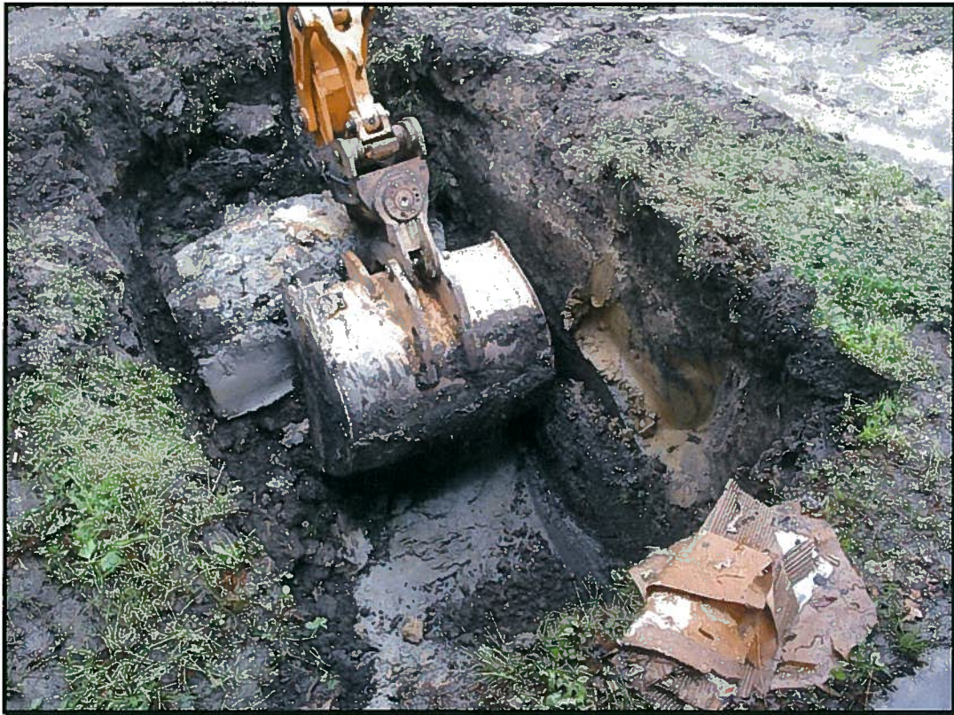
UST TT-2610 soil removal activities
