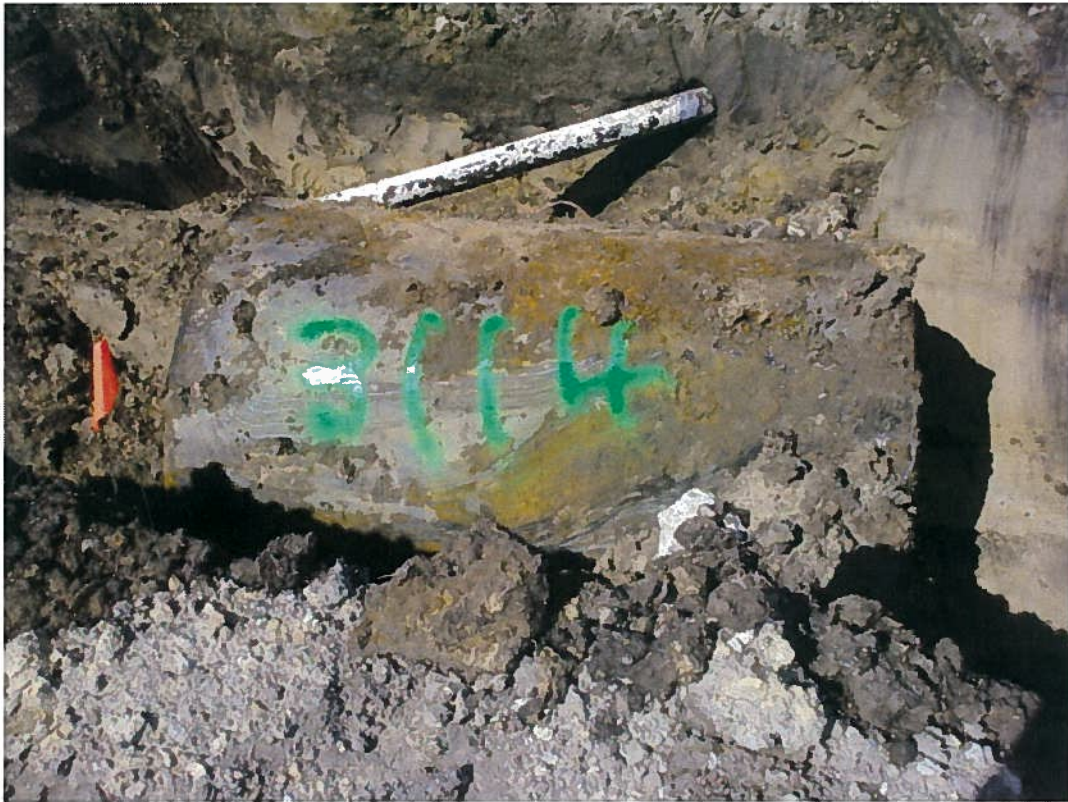
UST TT-3114 prior to removal
