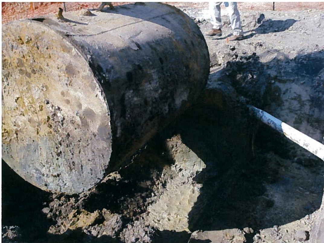
UST TT-3114 during removal activities
