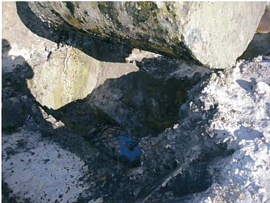
UST TT-3145 during removal activities
