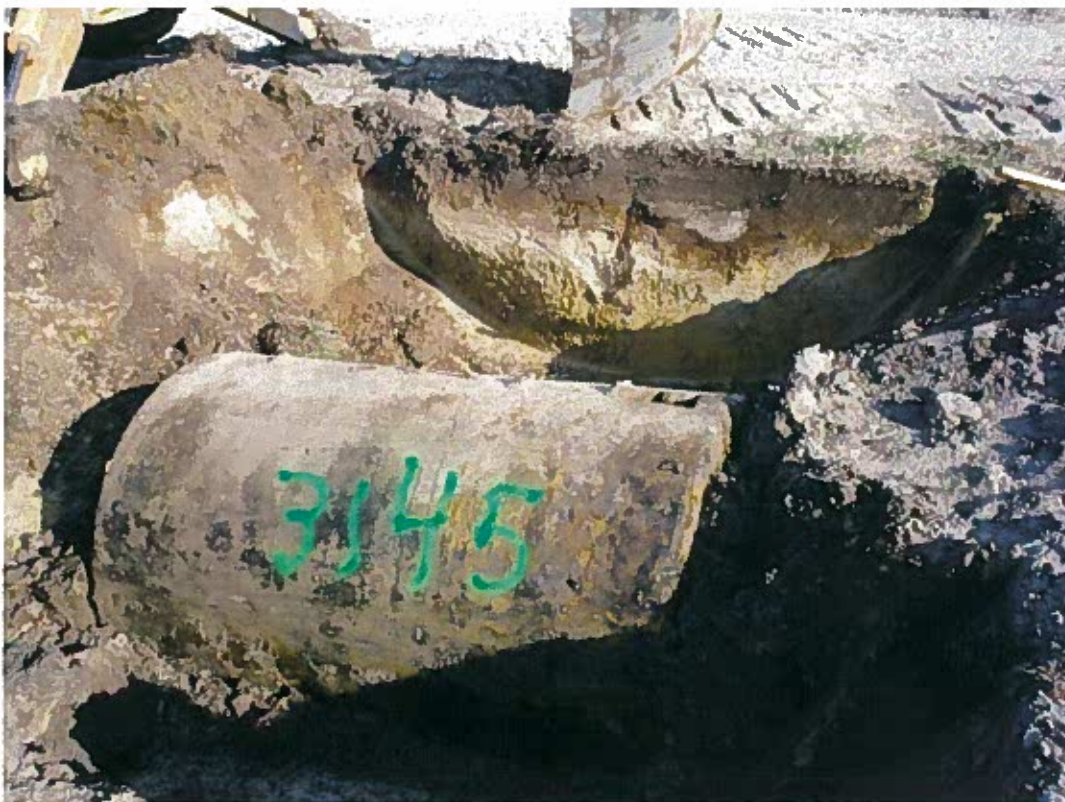
UST TT-3145 prior to removal with access hole
