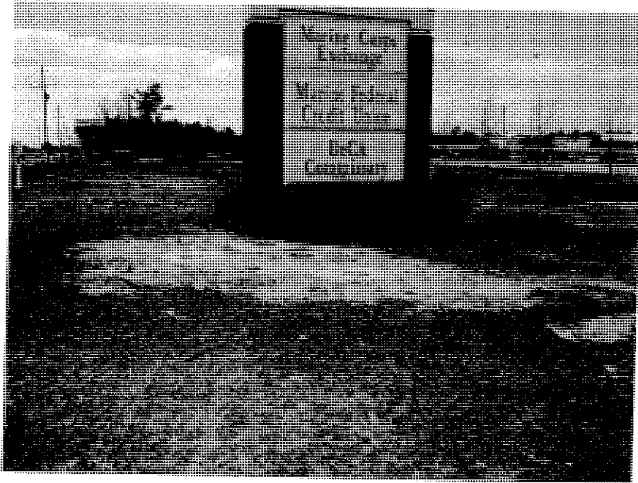
Holcomb Boulevard Excavation Restored to Original Grade
