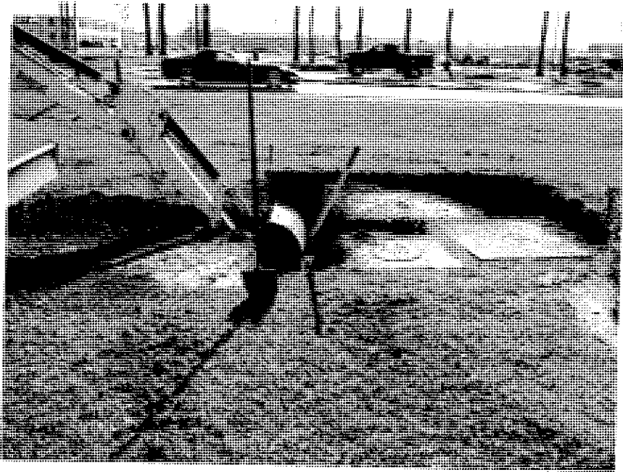
Holcomb Boulevard Initial Excavation
