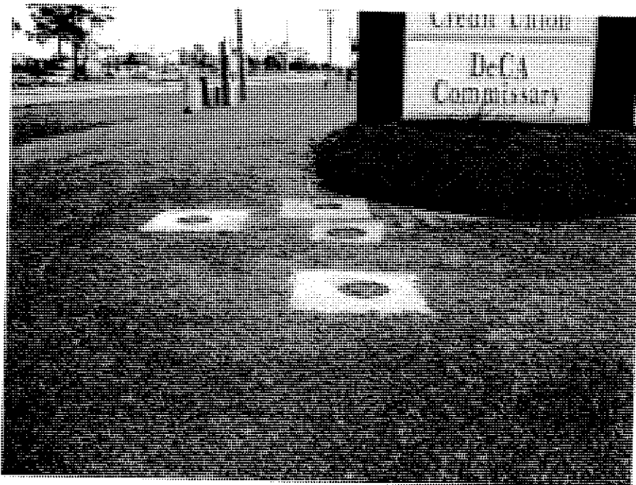
Holcomb Boulevard Excavation Area
