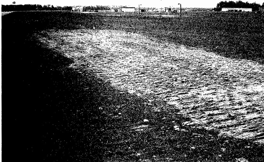
Completed excavation with backfill
