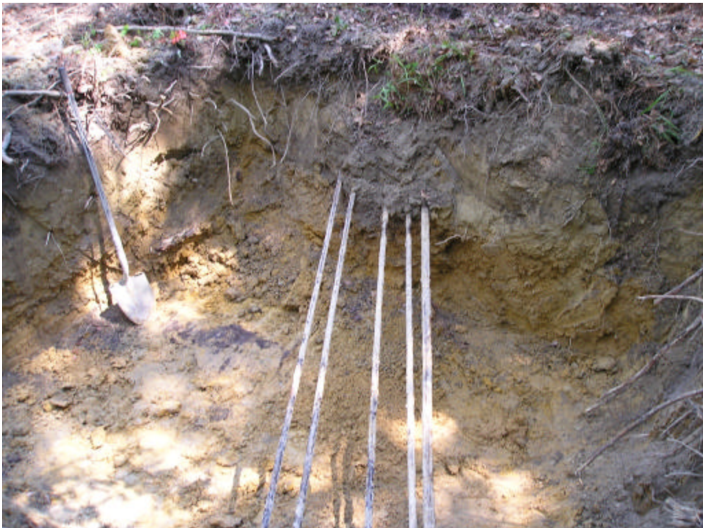
Excavation with Exposed Utility Lines (looking north)
