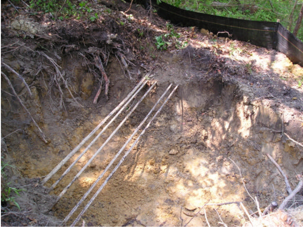
Excavation Looking South
