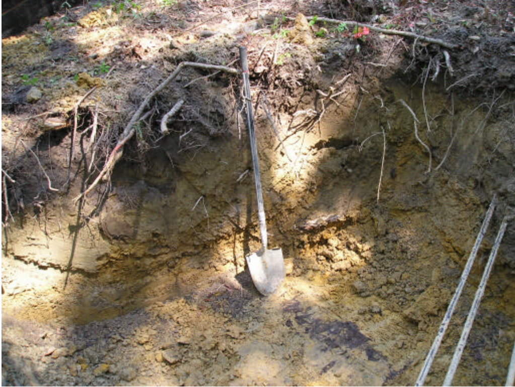
Excavation Approximately 4 Feet Deep
