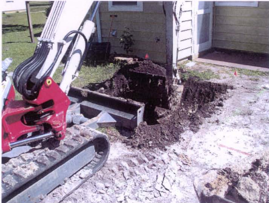
House pp-3350 Excavation
