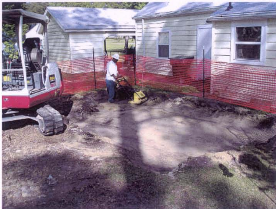
House pp-3326 Backfil
