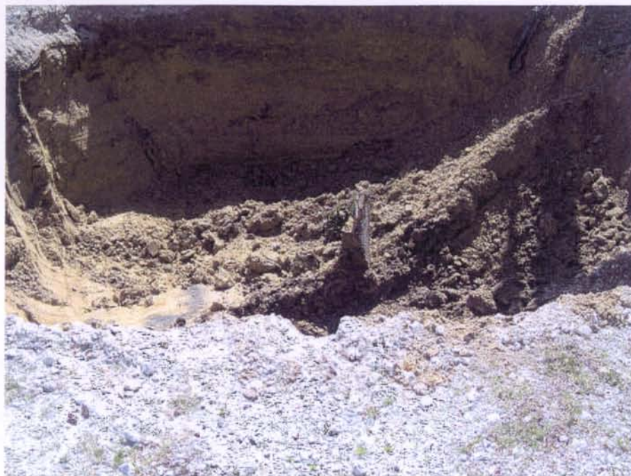
Building M-230 Excavations
