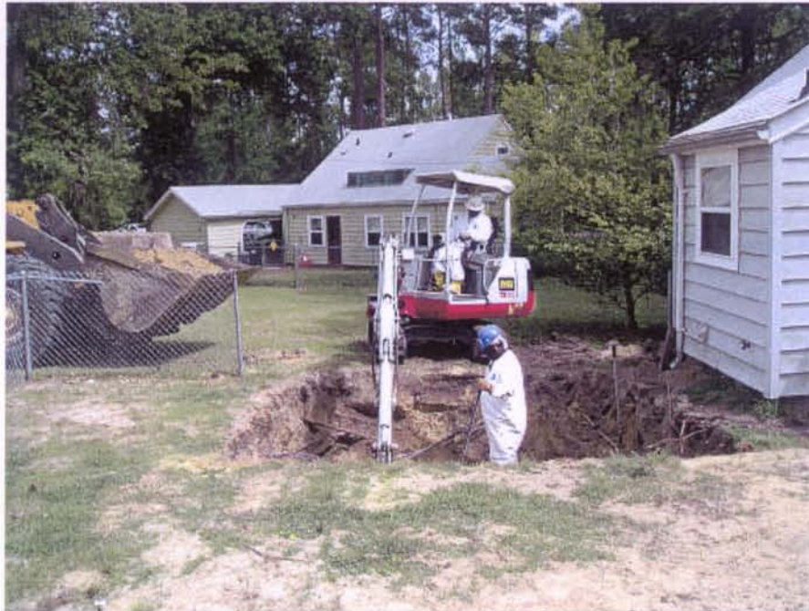
House pp-3330 Excavation
