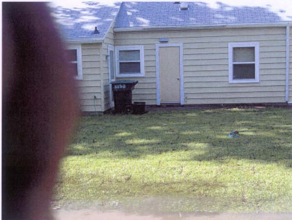
House pp-3350 Final
