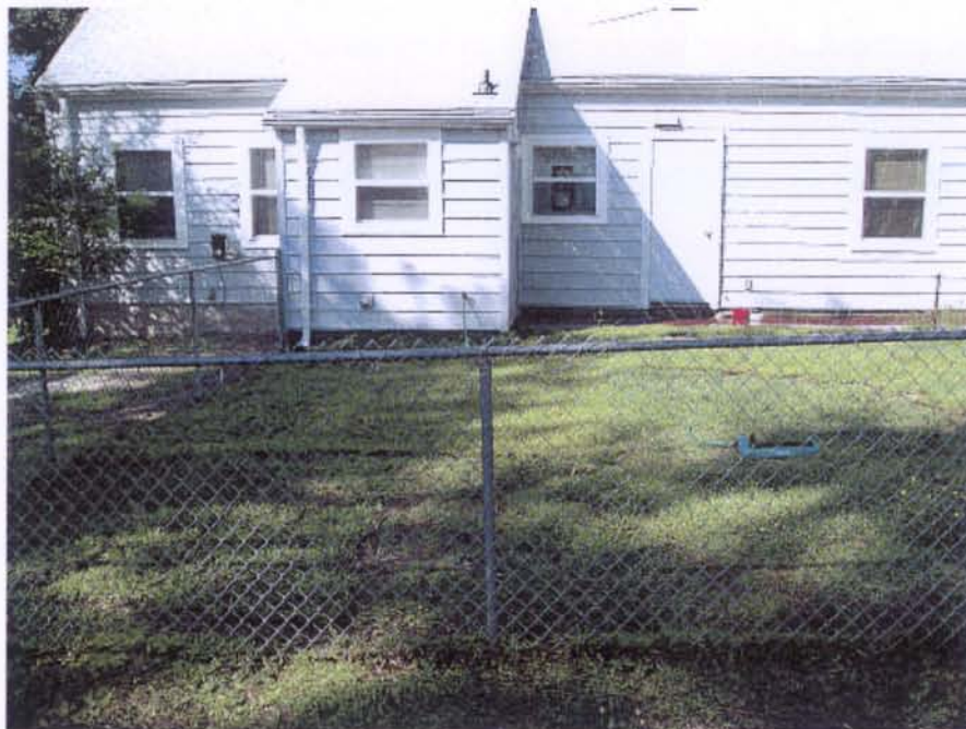
House pp-3330 Final
