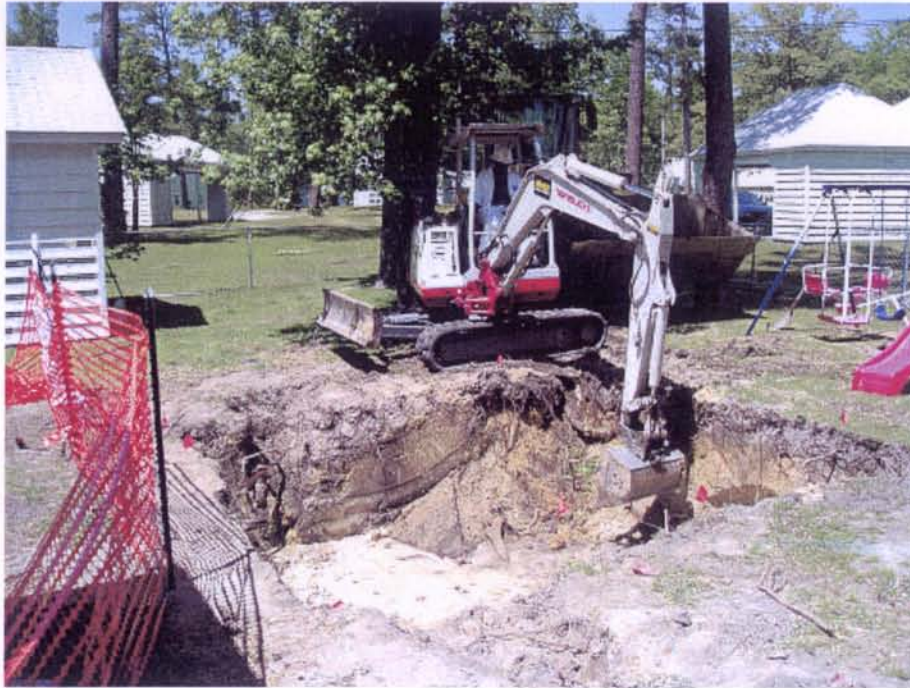
House pp-3332 Excavation
