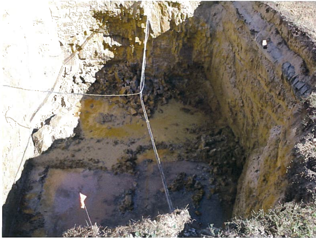
M-234 Excavation with Utilities
