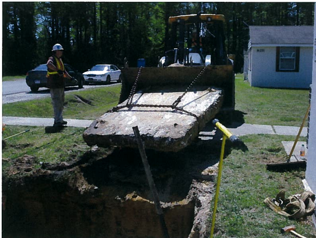
Removal of the Concrete Anchor Pad from M-234 Basin
