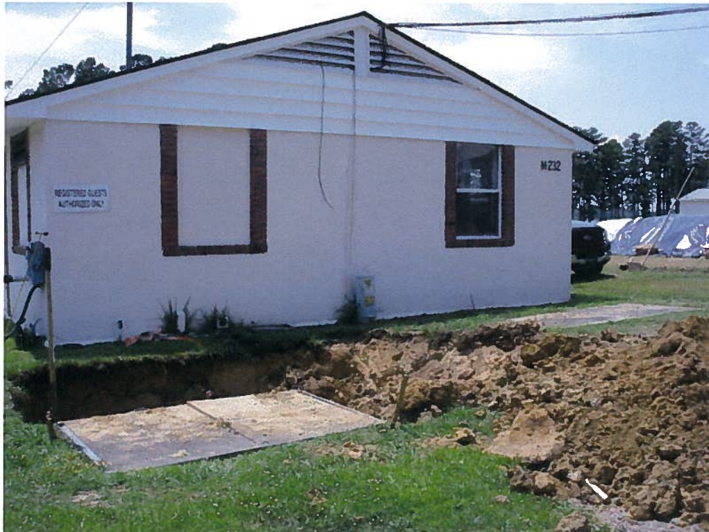
Start of M-232 Excavation Activities
