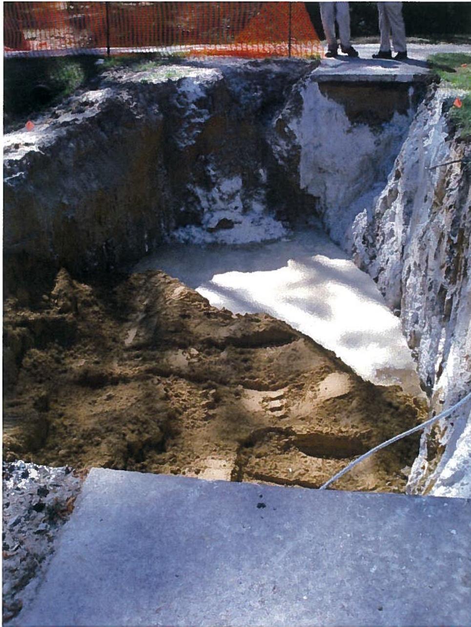
Application of ORC and Beginning of Backfilling at M-236
