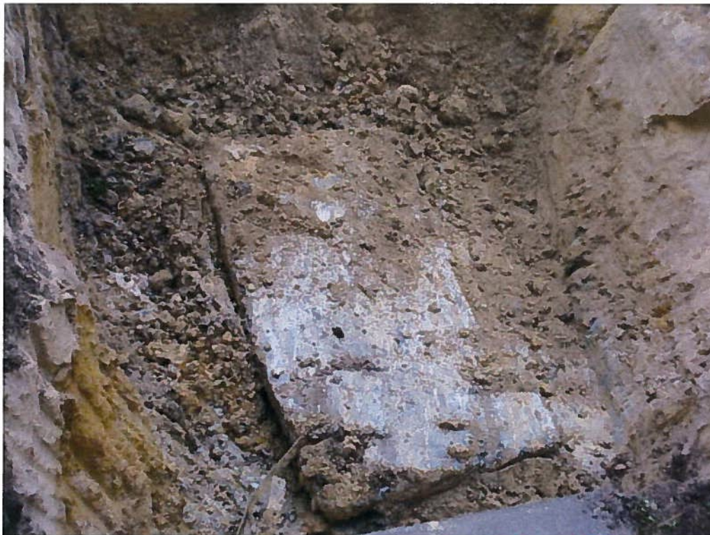
Concrete Anchor Pad at Bottom of M-236 Basin before Removal
