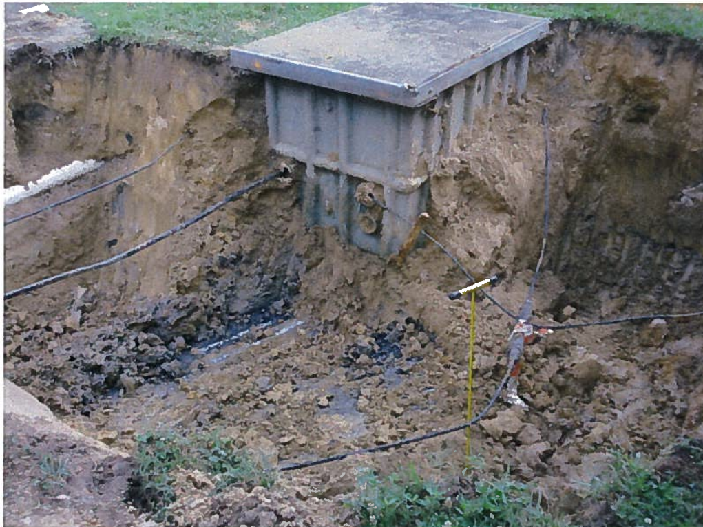
Exposing Communications Box and other Utilities within Excavation
