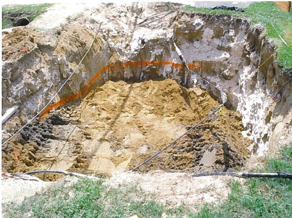
Partial Backfilled M-232 Excavation
