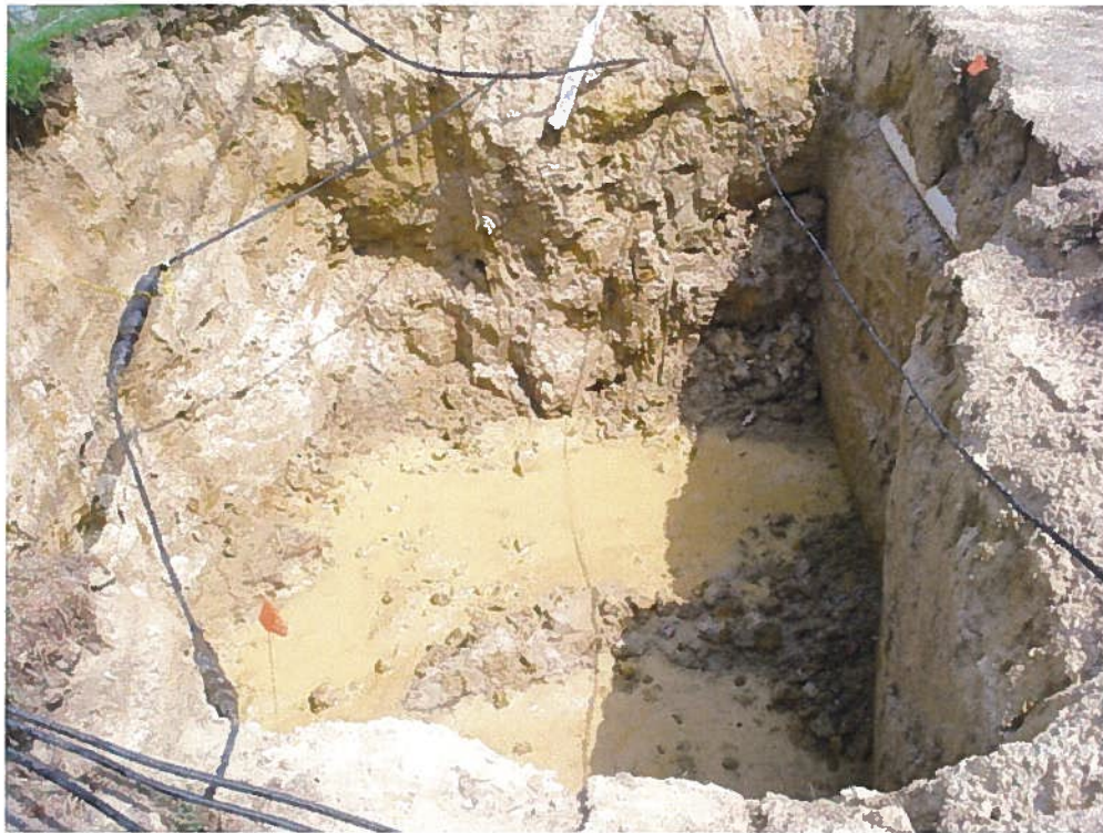
Bottom of M-232 Excavation after Concrete Pad Removal
