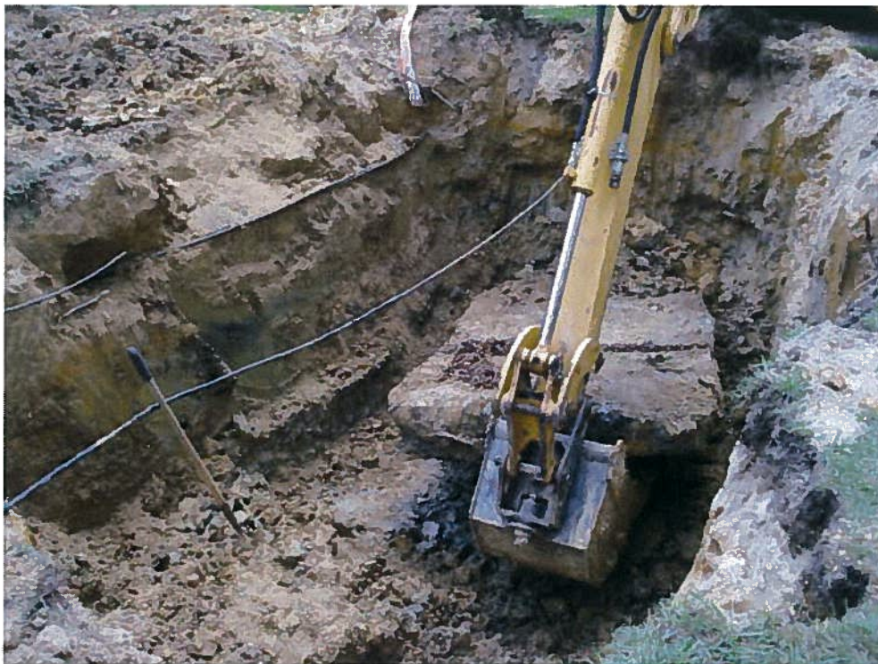
M-233 Excavation and Removal of Concrete Anchor Pad
