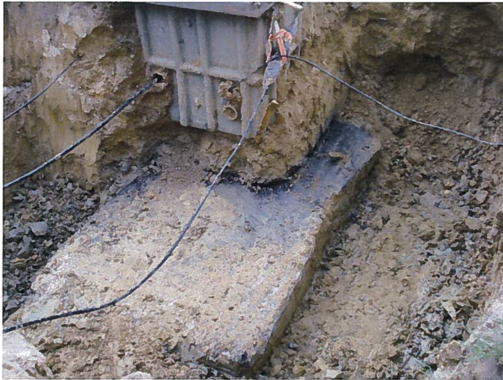
Large Concrete Anchor Pad at Bottom of M-232 Basin
