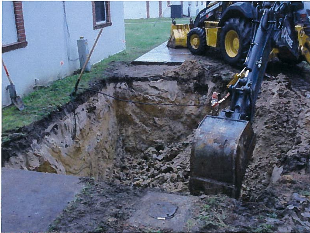
M-236 Excavation Activities
