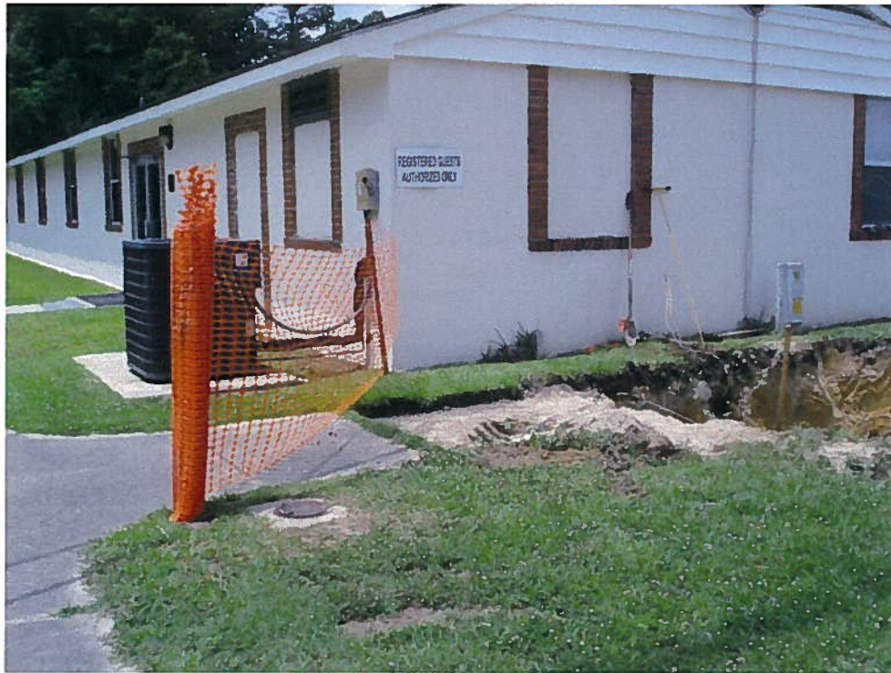
Start of M-233 Excavation Activities
