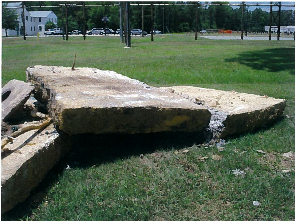
M-232 Concrete Anchor Pad after Removal from Basin
