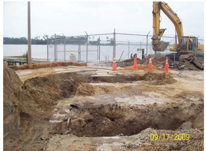
Photograph 4: A view towards the southwest looking at the excavation of line set A. The original trench is to the left; however, the line set curved and perpendicular trenches had to be cut to retrieve the line due to monitoring wells in the area.
