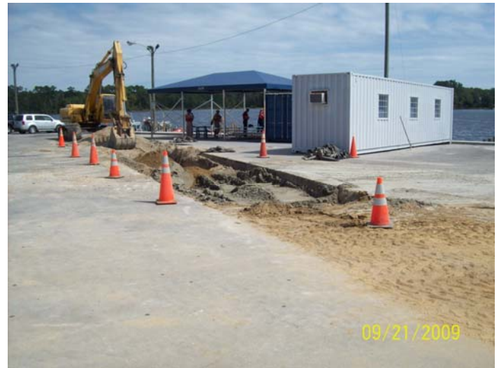
Photograph 6: A view towards the southeast looking at the final excavation of line set E towards the bulkhead.
