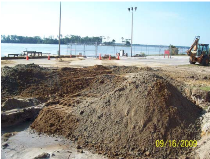
Photograph 5: A view towards the southwest looking at the initial excavation pit being backfilled with clean silty fine-grained sand.
