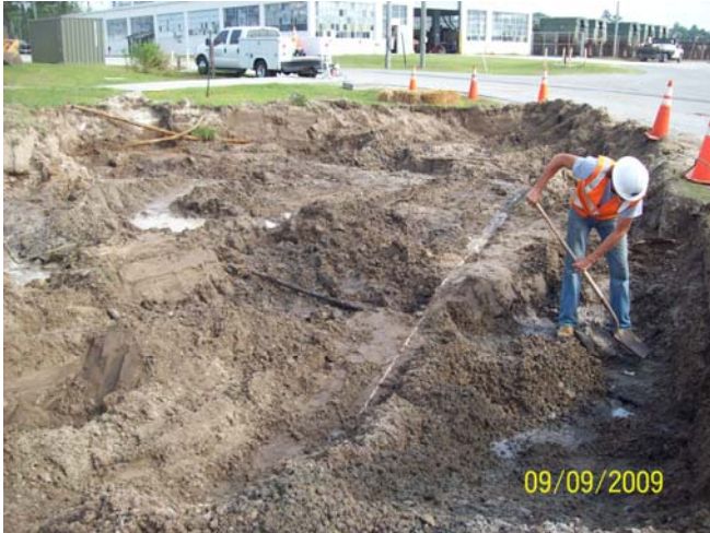
Photograph 1: A view towards the northeast looking at the exposed 2 inch PVC pressurized water line.
