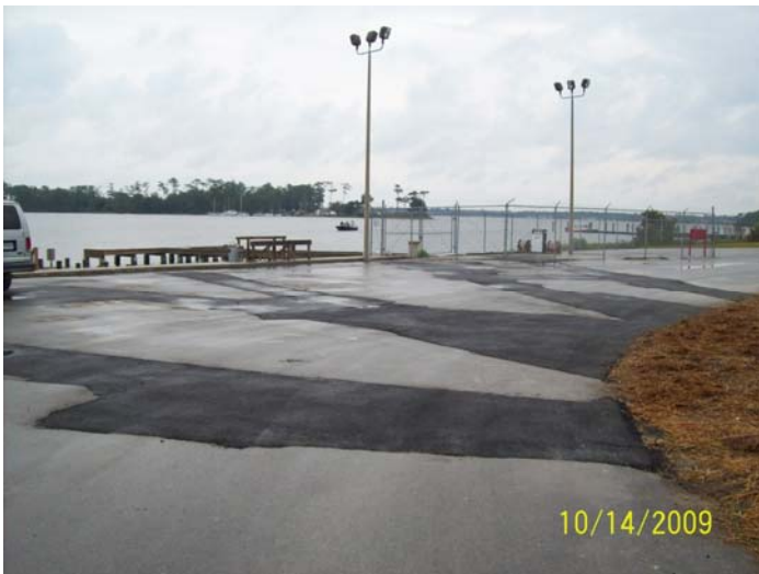
Photograph 7: Asphalt pavement looking toward the New River.
