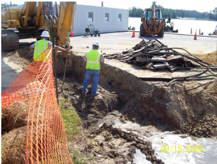
Photograph 3: A view towards the southeast looking at the initial excavation of line set E. Note the storm drain line which lies below the fuel lines.
