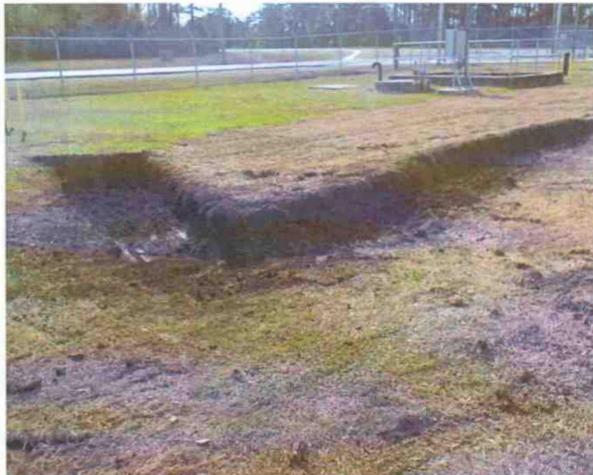
Campbell Street Fuel Farm Release Dig 1 of 3 - Picture 6 of 6
