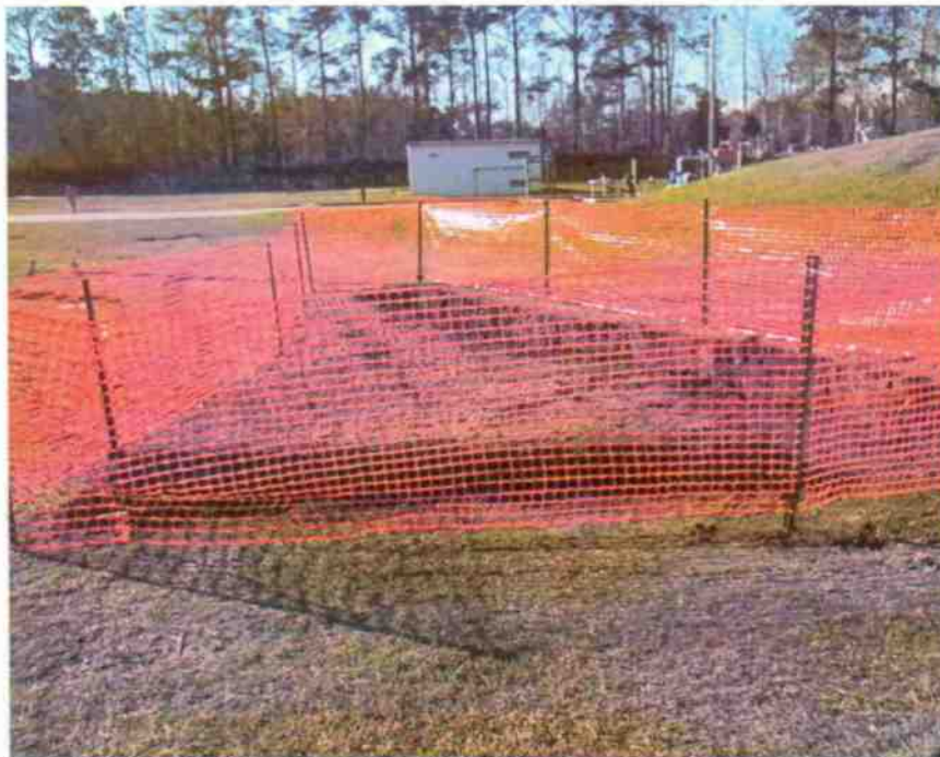
Campbell Street Fuel Farm Release Dig 1 of 3 - Picture 4 of 6
