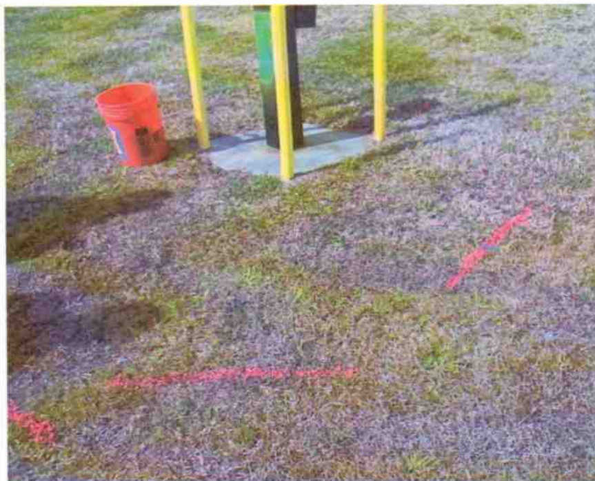
Campbell Street Fuel Farm Release Dig 1 of 3 - Picture 2 of 6
