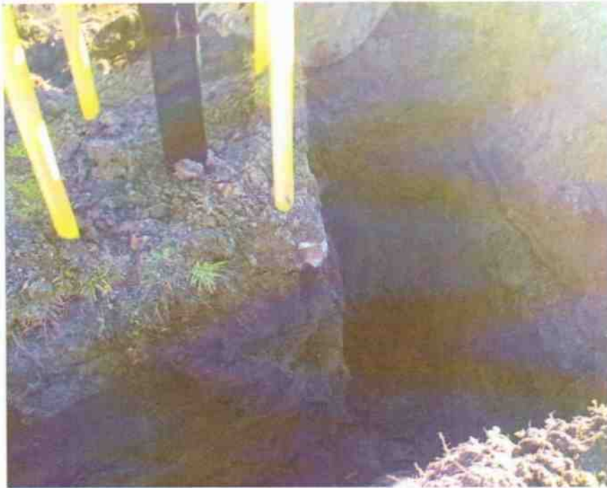
Campbell Street Fuel Farm Release Dig 1 of 3 - Picture 3 of 6
