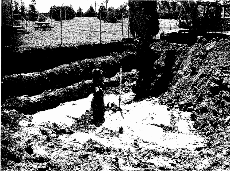
AS840 during Excavation
