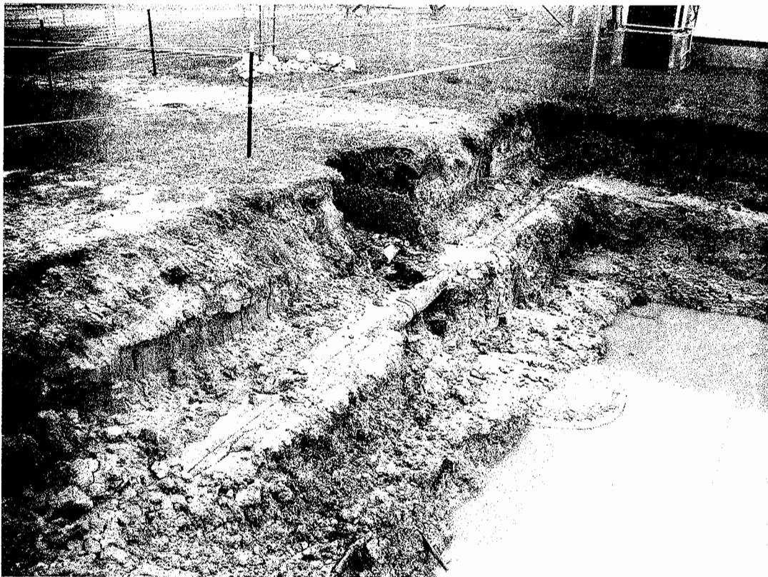
Utility Line along North Sidewall
