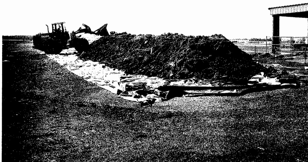
Impacted Soil Stockpiled Just Prior to Disposal
