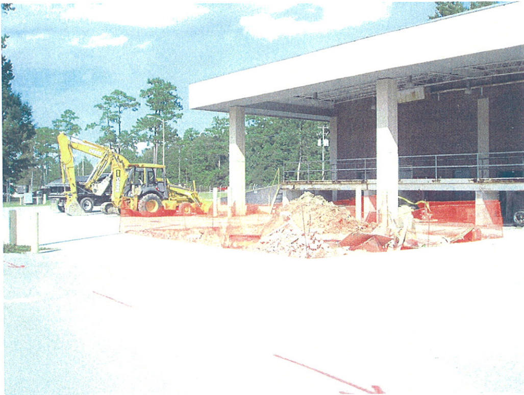
Building AS-4159 OWS and UST Location
