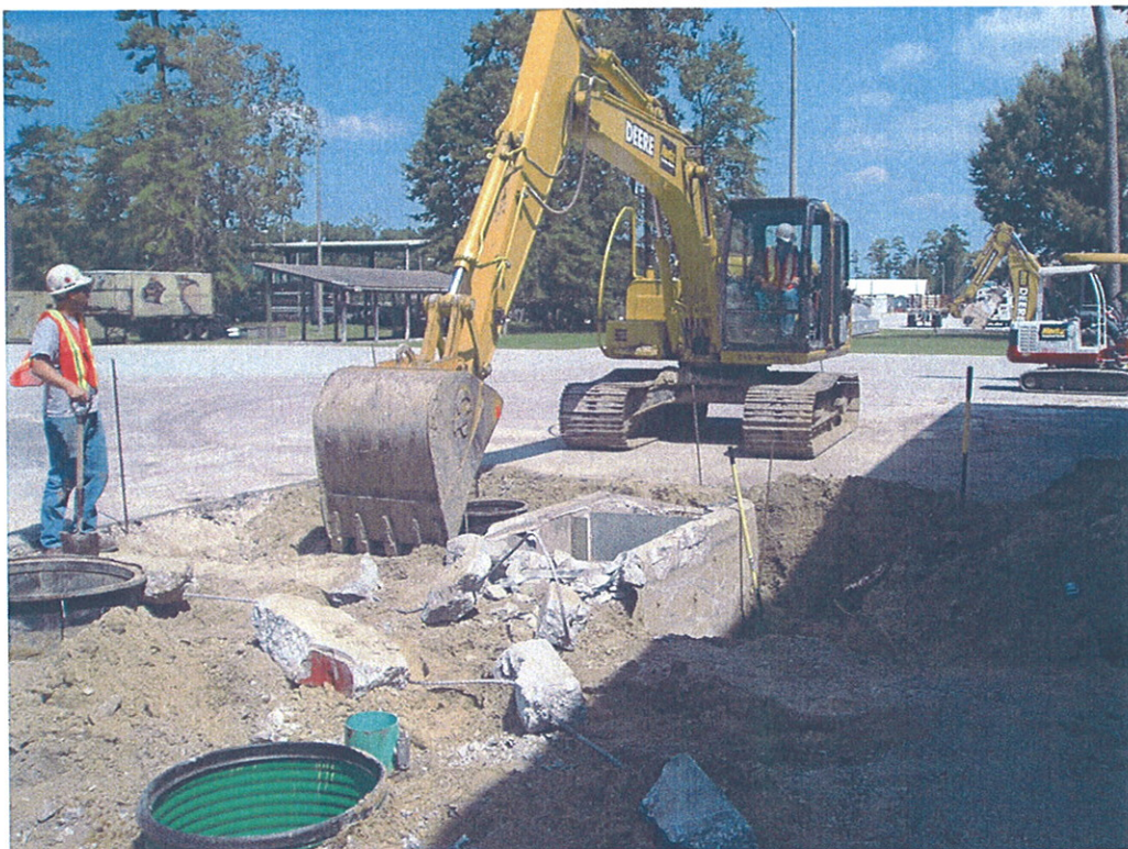
Building AS-4159 OWS Removal
