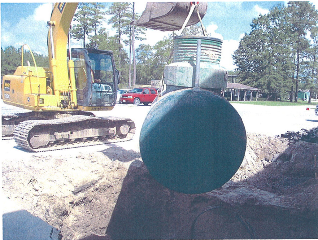
Building AS-4159 UST Removal
