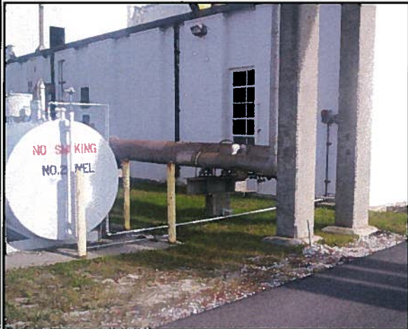
Looking Northeast – Towards Building AS-4151
