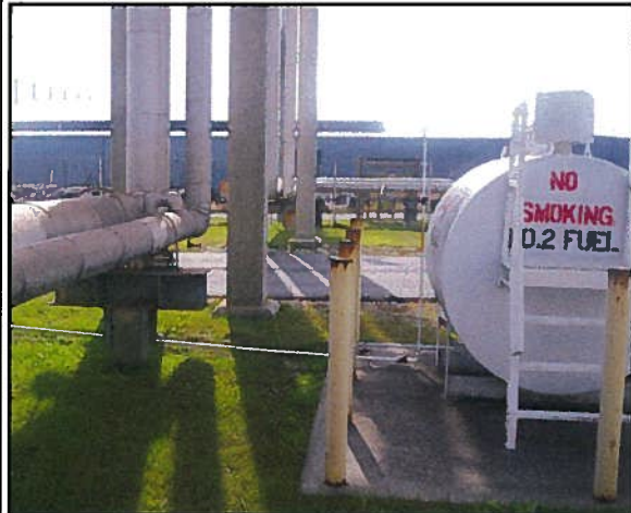
Looking South – Away from Building AS-4151
