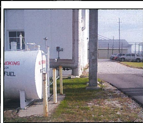
Looking East – Along southern side of Building AS-4151
