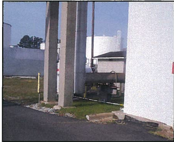
Looking Northwest – Towards Southwest corner of Building AS-4151
