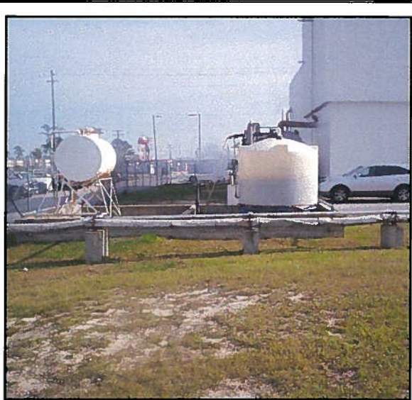
Looking East – Towards Building AS-4151
