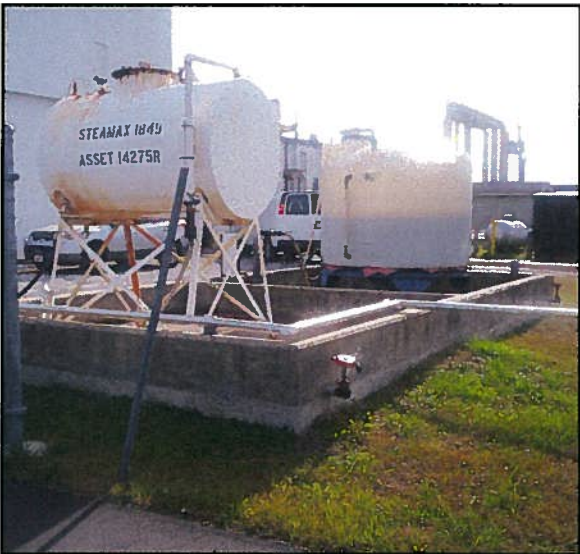
Looking South-Southeast – Toward Building AS-4151
