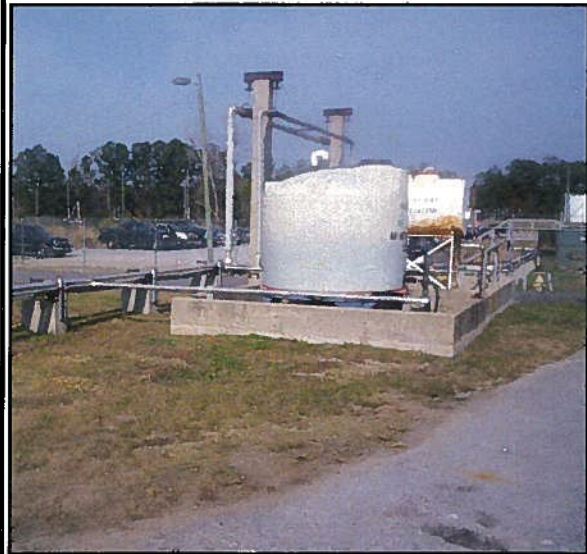
Looking North – Away from Building AS-4151
