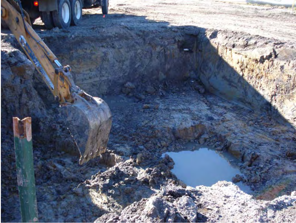
UST TT-3026 – Tarawa Terrace –Tank Pit Re-Excavation Pic #1 30Oct08
