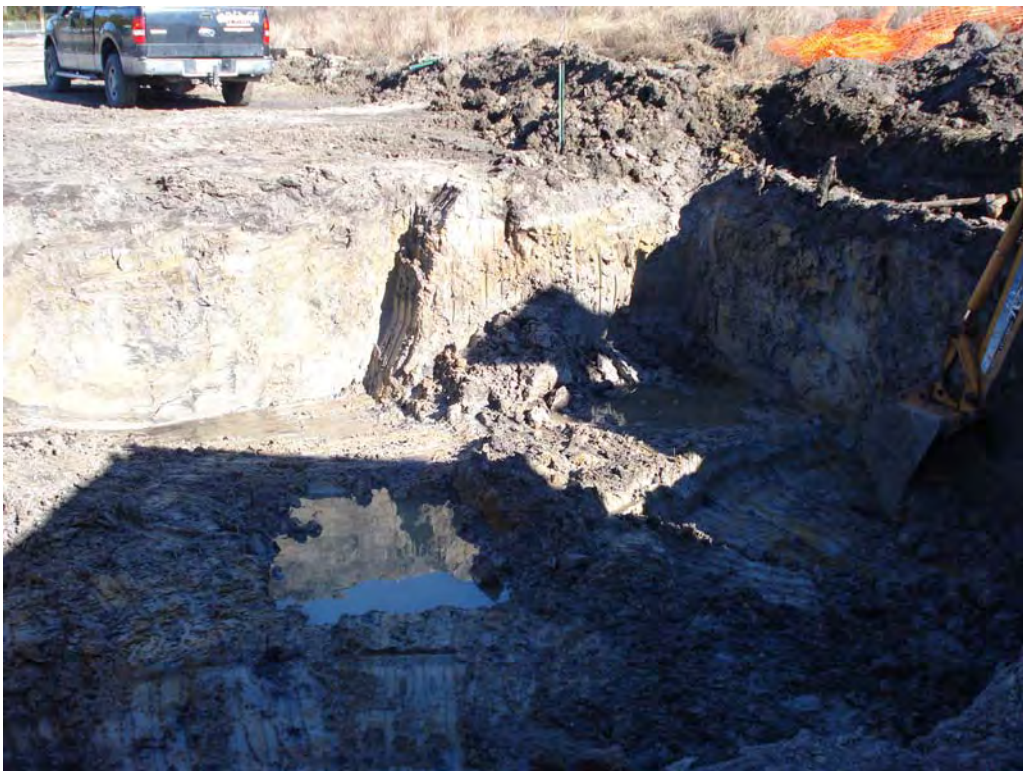
UST TT-3026 – Tarawa Terrace –Tank Pit Re-Excavation Pic #2 30Oct08
