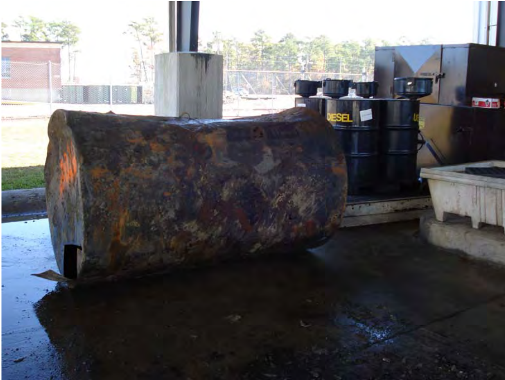
UST TT-3026 – Tarawa Terrace –Tank Topside Pic #1 24Oct08
