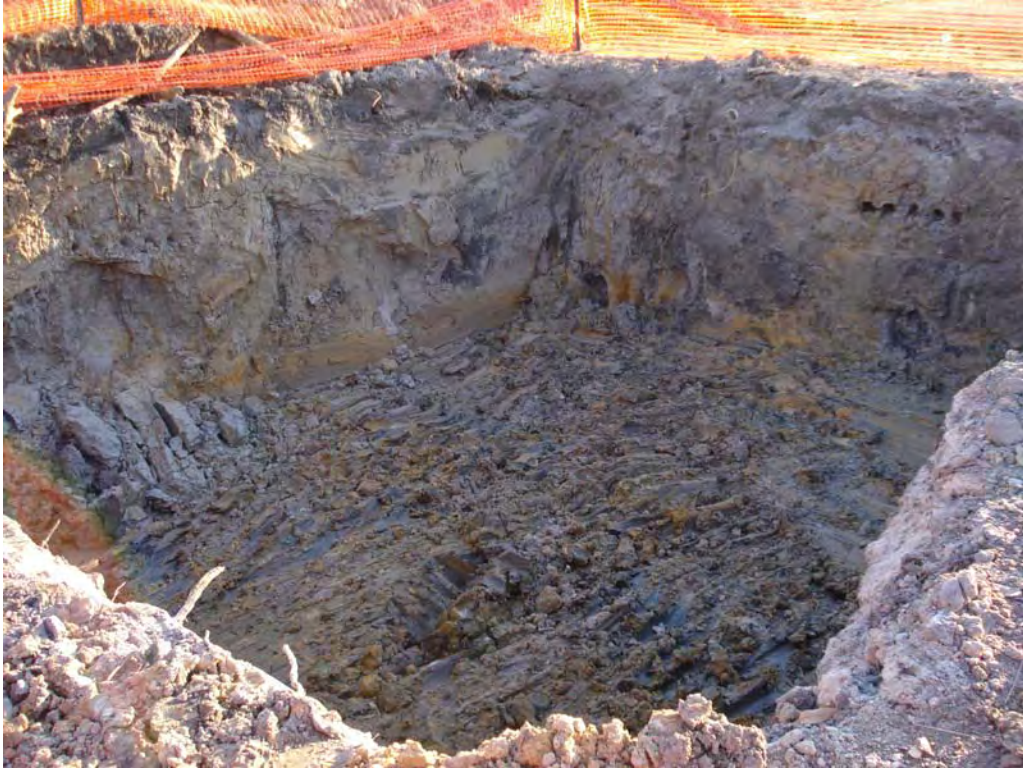
UST TT-3026 – Tarawa Terrace –Tank Pit Final Excavation Pic #1 21Nov08
