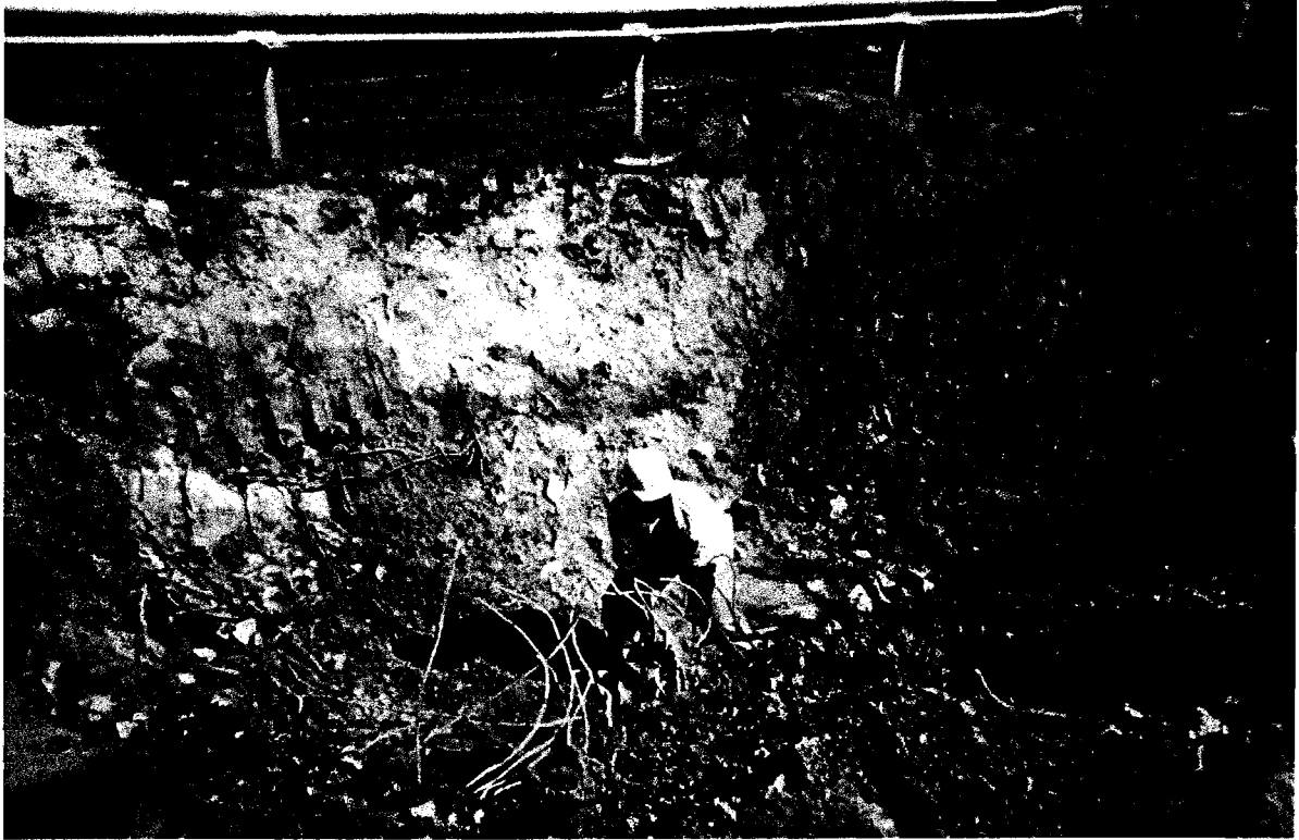
Photo 9 Partially backfill and cutting concrete re-bar prior to sampling at UST bottom
