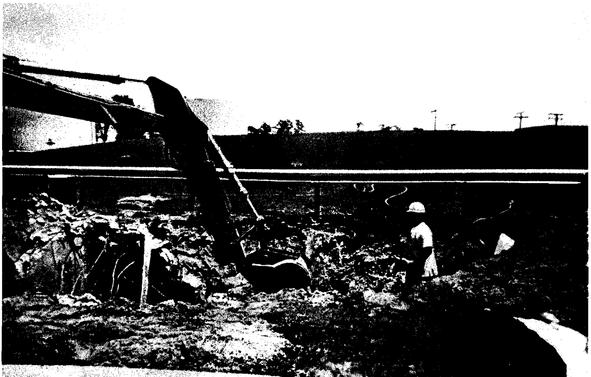
Photo 8 Concrete UST demolition ---- Note landslides occur around supports of a fuel pipe
