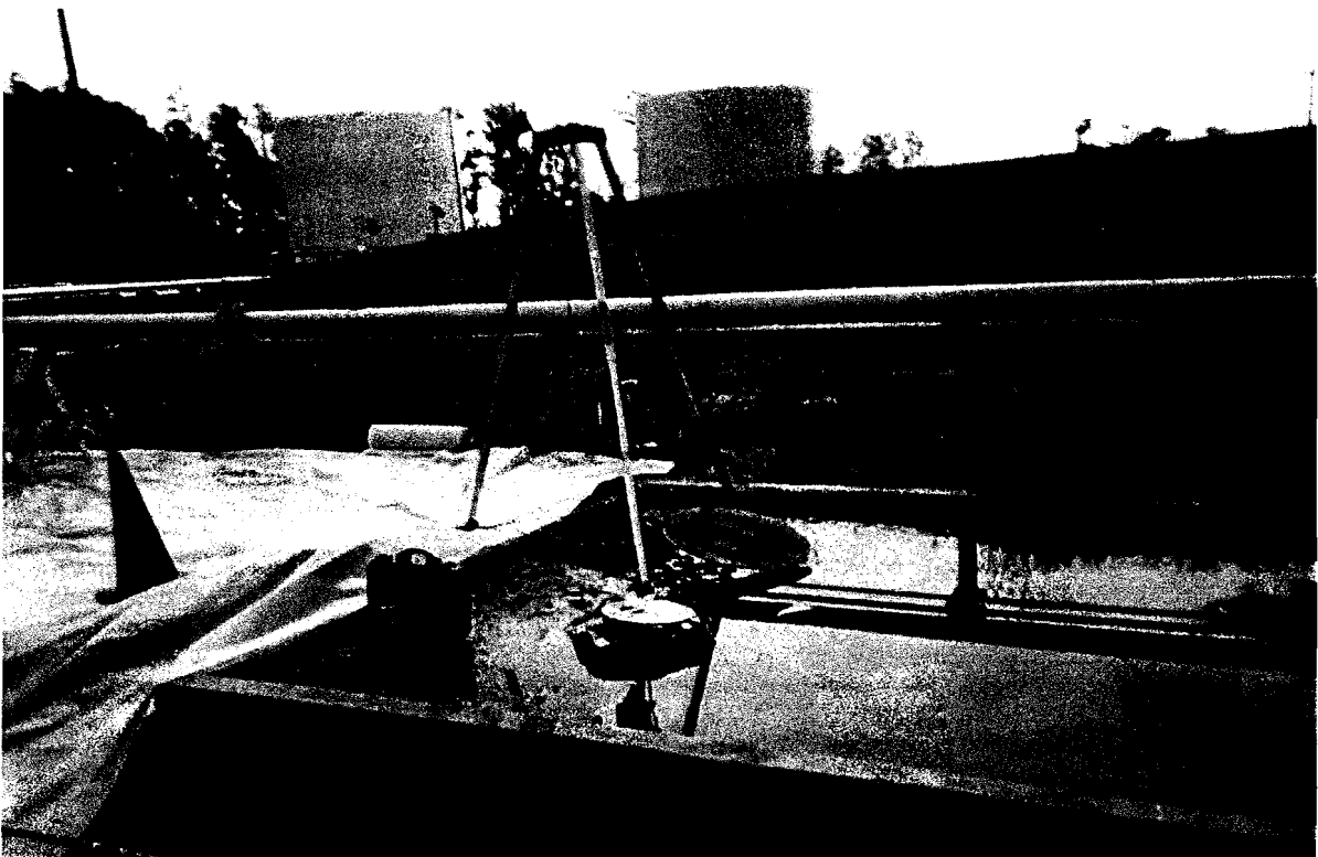
Photo 2 Set-up for UST cleaning ---- Confined space entry
