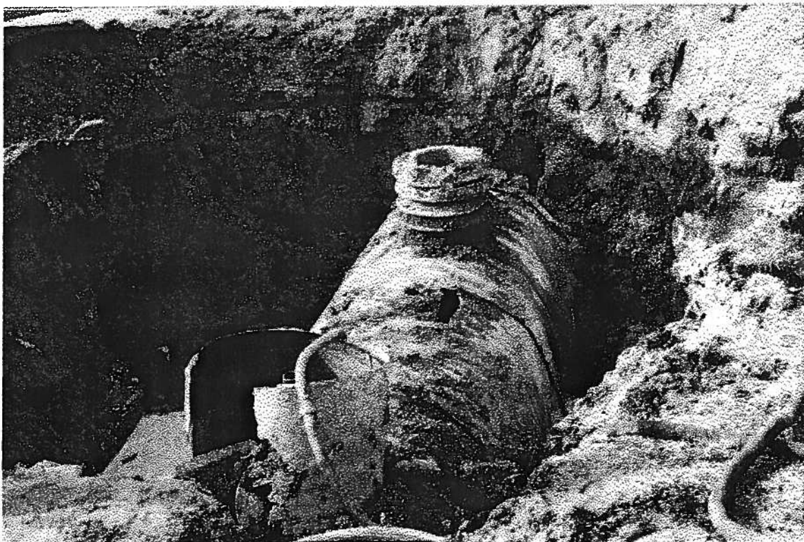
Photo 7 The fiberglass UST exposed. Note ground water in excavation pit
