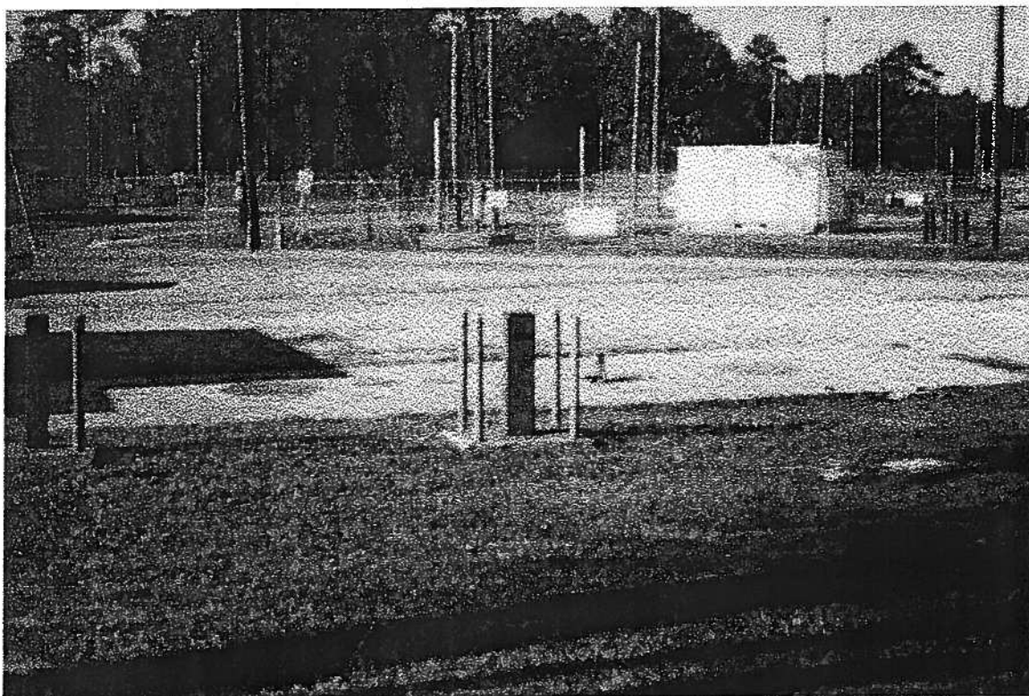
Photo 3 Site view prior to excavation activities
