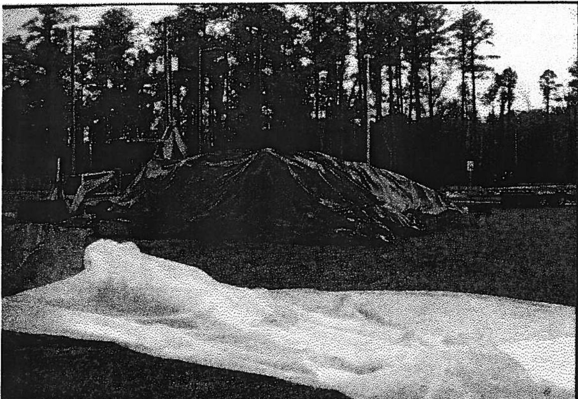
Photo 12 The soil excavated is properly stockpiled
