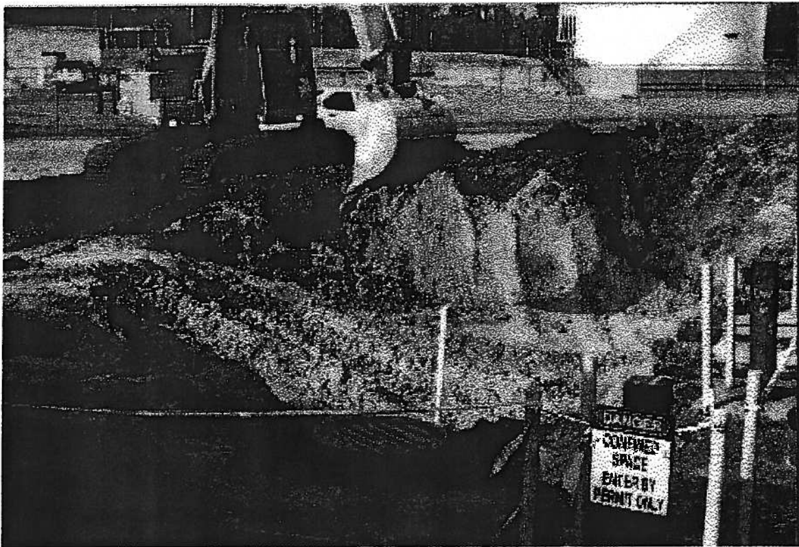
Photo 9 The excavation is backfilled with clean sand
