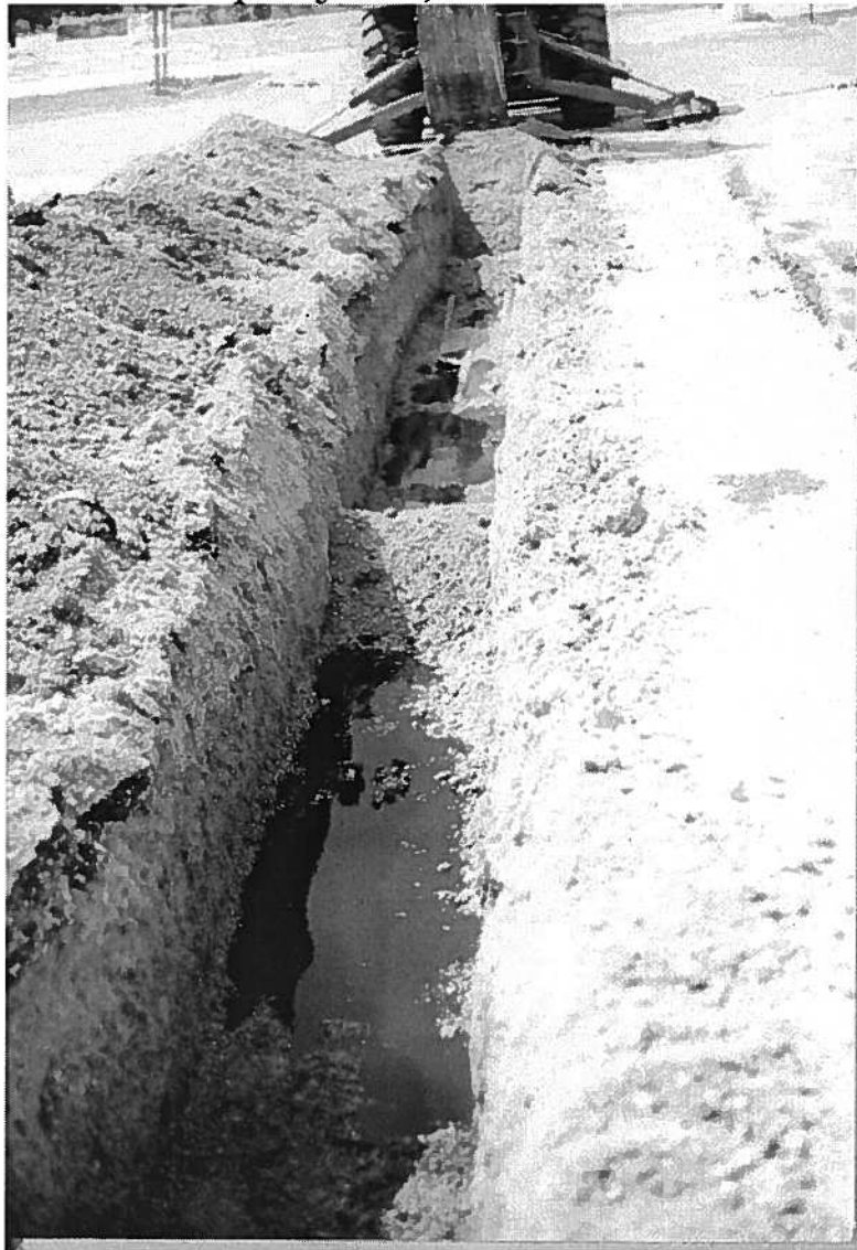
Photo #6 Free product in fuel supply line trench
