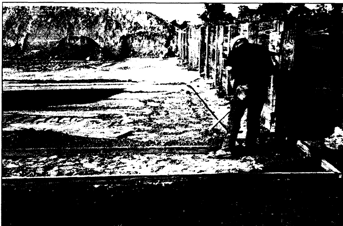
Photo 10. Forming Gravel Walkways
