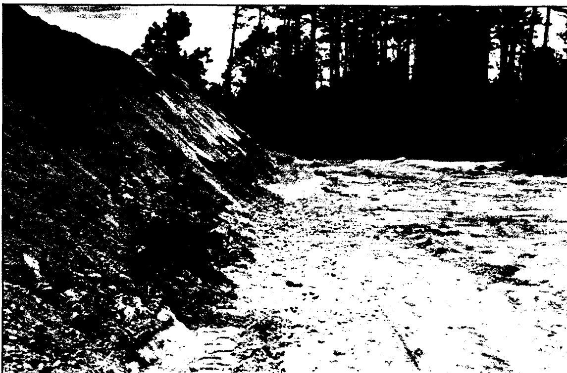
Photo 9. Gravel-Lined Drainage Channel at the Base of the Completed Berm
