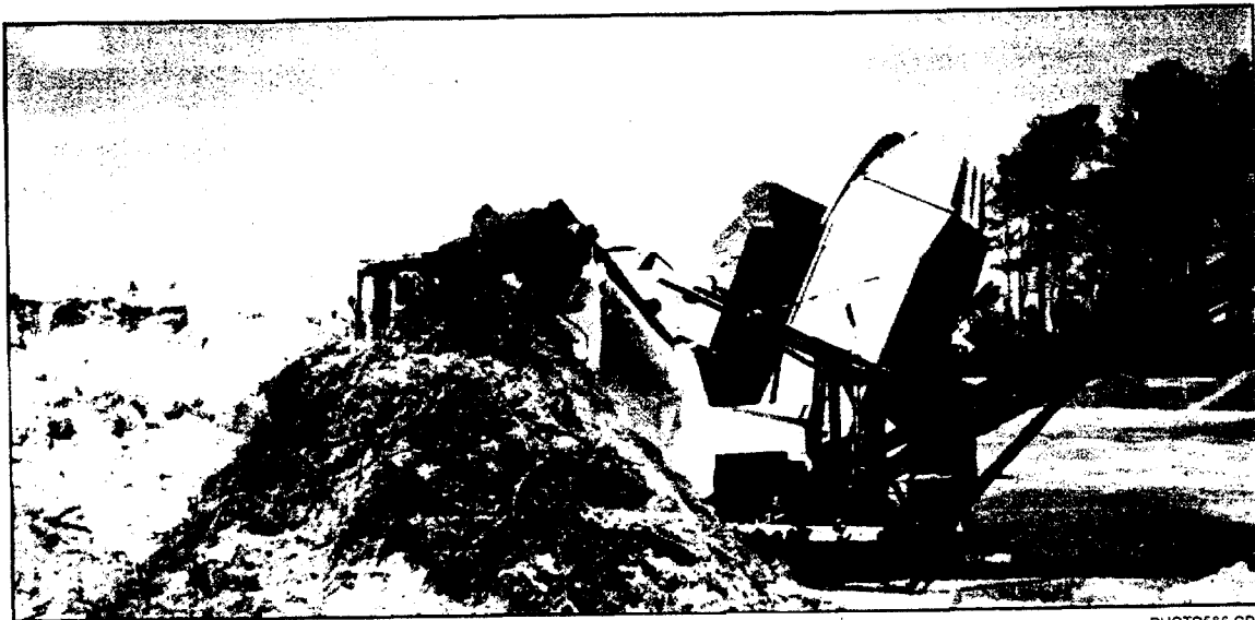
Photo 5. Organic Debris Removed from Lead-Bearing Material Prior to Recycling
