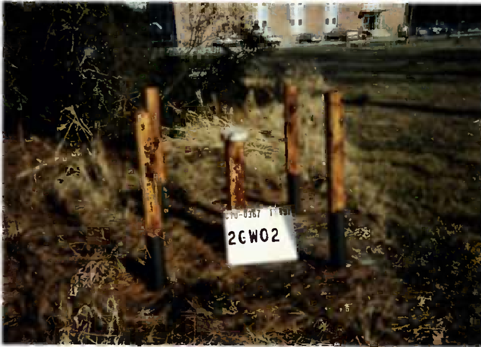
Figure 3-3 Shallow monitoring well 02-GW02 was constructed during the 1984 Confirmation Study. The well had begun to exhibit signs of subsurface deterioration.
